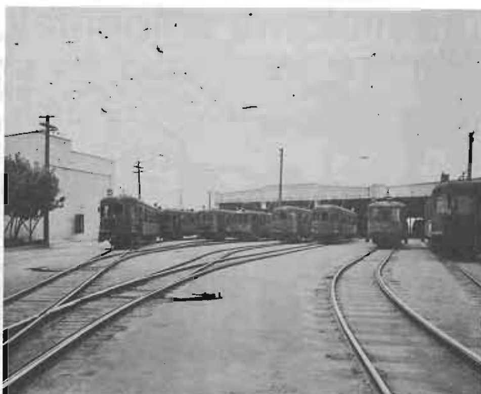
Tracks and power lines crisscross the yard at Division 5 in this mid-1930s view of what was then a Los Angeles Railway (LARY) operating facility. The squat concrete building to the left was a power station. It was replaced in 1978 by a modern train room. The "M" on the cars' headsign stood for the Monita Line which is today Line 7. With its new transportation building, modern bus washing and fuel facility and soon-to-be remodeled maintenance structure, Division 5 today is home to nearly 600 bus operators who use the 300 buses assigned to the division to work 19 lines serving the South Central portion of the city, downtown Los Angeles, Hollywood, Whittier, Norwalk, Marina del Rey, Manhattan Beach and Los Angeles International Airport. Approximately 130 mechanics staff the facility, which is one of the District's largest and busiest.
