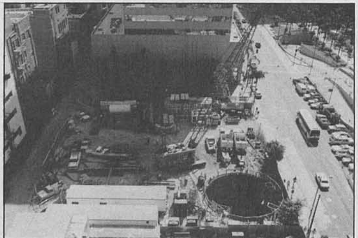
Aerial view of the construction site at 5th and Hill Streets.
