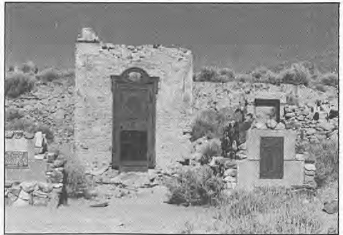
The remains of the Bodie Bank after the disastrous fire of 1932.
