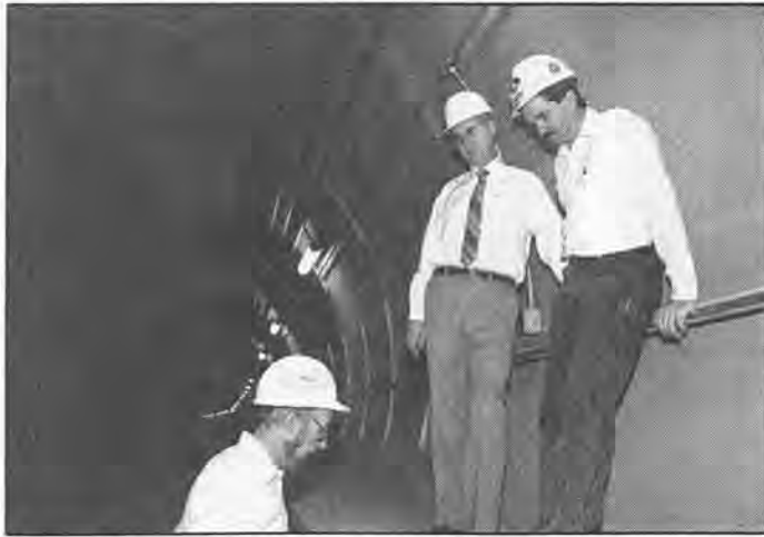
Albert H. Perdon (center) along with RCC Chief Executive Officer Ed McSpedon (right) listen to Resident Engineer Bob Griffith at the A171 site inside the Westlake/MacArthur Metro Rail tunnel.
