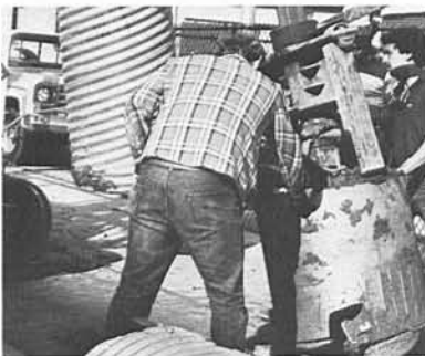
Core samplings indicate favorable tunneling conditions along entire 18-mile subway route.
