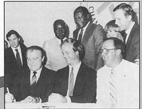
Local leaders and Ralph Stanley (center) witness historic MOS-1 construction contract signing.
