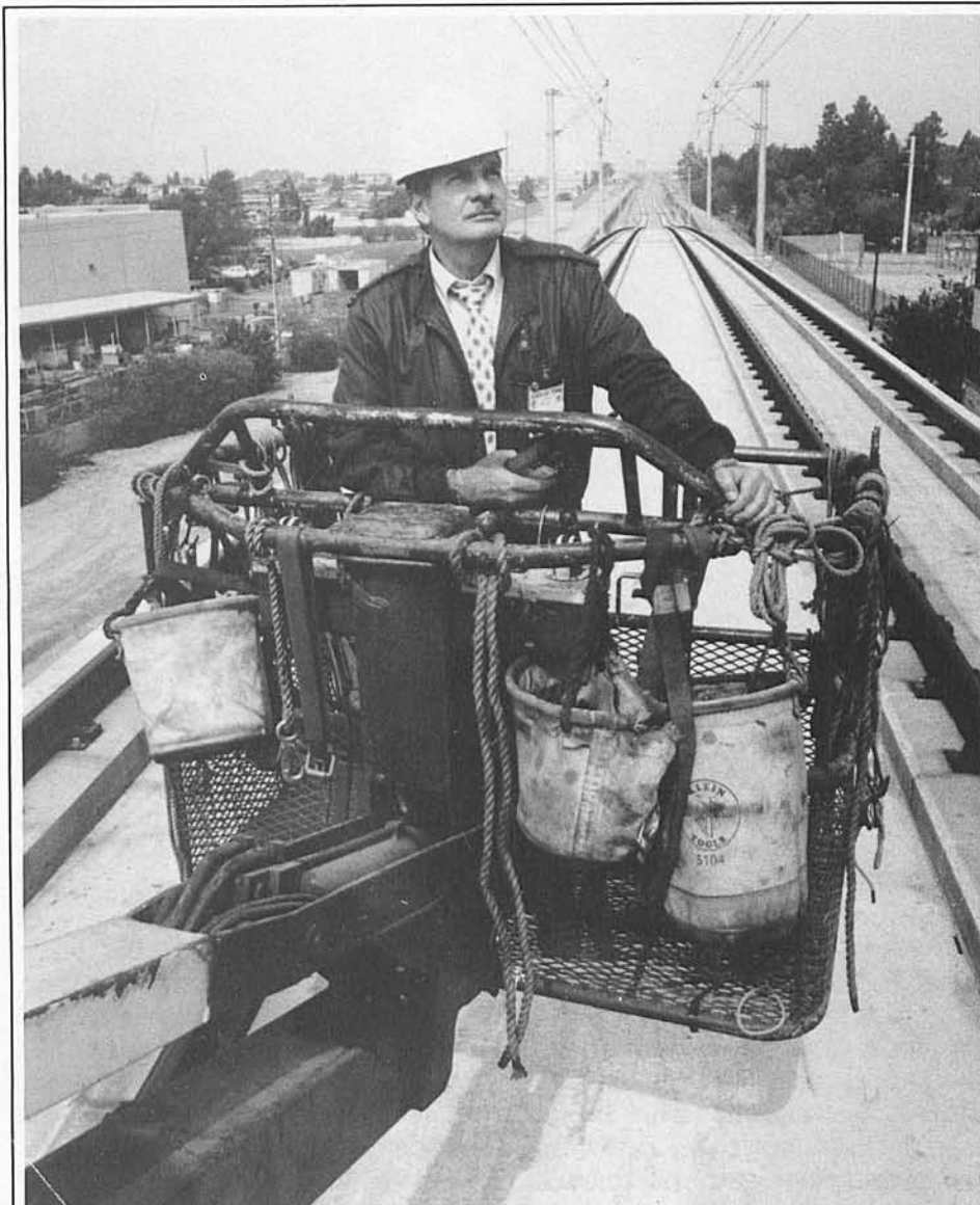
HIGH WIRE ACT — Railroad expert Walter "Bud" Moore checks the aerial cables that will propel the Metro Blue Line train along 22 miles of track between Los Angeles and Long Beach. The master electrician, who brings to RTD years of expertise with the Chicago Transit Authority, is rail facilities superintendent for the Blue Line, which RTD is scheduled to begin operating July 14.
