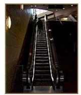
**Segment 1 Metro Red Line Stations** (Jan. 28) Fifteen of the 42 escalators in the Segment 1 Metro Red Line stations have been upgraded with bright, new fluorescent lighting. The new lights meet state safety codes that require illumination for escalator steps.
