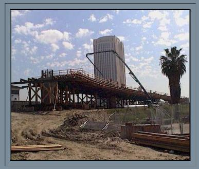
(April 2) Just east of Union Station, the arm of a crane reaches over the unfinished Pasadena Blue Line ramp to pump concrete into a wooden form. Construction on the rail line also is under way in Old Pasadena and on the section of the line that will pass beneath Figueroa Street, north of the Pasadena Freeway. Photo By NATE BAGUIO
