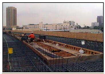
Since this photo was taken of workers installing reinforcing steel in early October, the concrete for the deck has been poured. This section from Union Station to North Spring Street in Chinatown is essentially complete.
