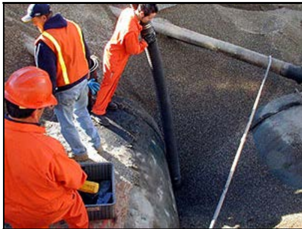
^ A crew excavates contaminated soil around a waste oil and chemical storage tank.
