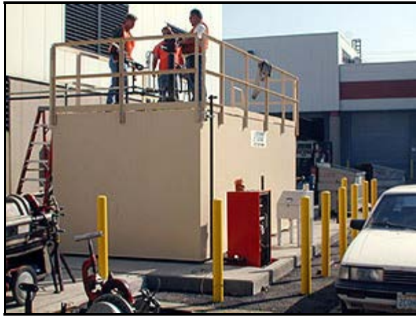
^ Workmen put the final touches on an aboveground diesel fuel storage tank at the RRC.
