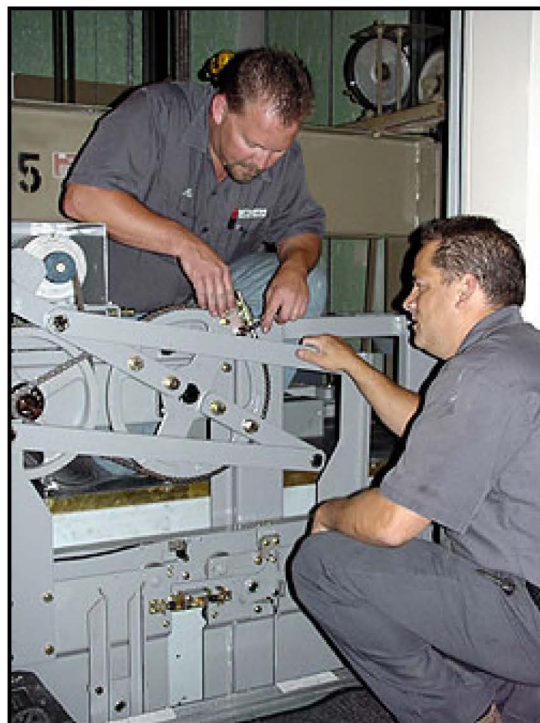
^ Mechanics Mike Mershon and Nick Trujillo of Mitsubishi Electric adjust a new heavy-duty door operator on an elevator in the low-rise bank at MTA Headquarters. Modernization of elevators in the high-rise bank is scheduled to start in July. PHOTO BY BILL HEARD.
