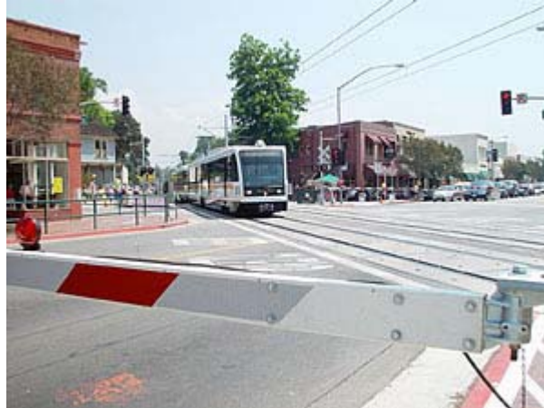
4-quad crossing gates guard Mission Station intersection.
