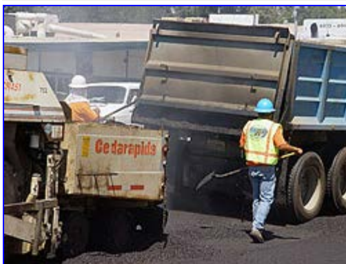
Steam rises from fresh asphalt as a paving machine lays a new road surface on Woodman Avenue near Oxnard Street in Van Nuys.
