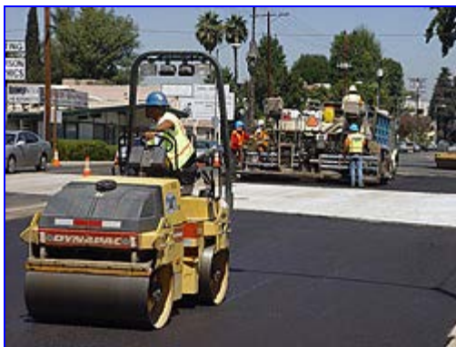
A compactor compresses the newly laid asphalt on the transitway at the Woodman Avenue crossing.
