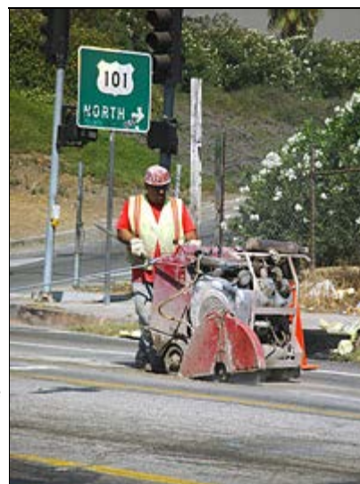
A construction worker maneuvers a pavement cutter along First Street
