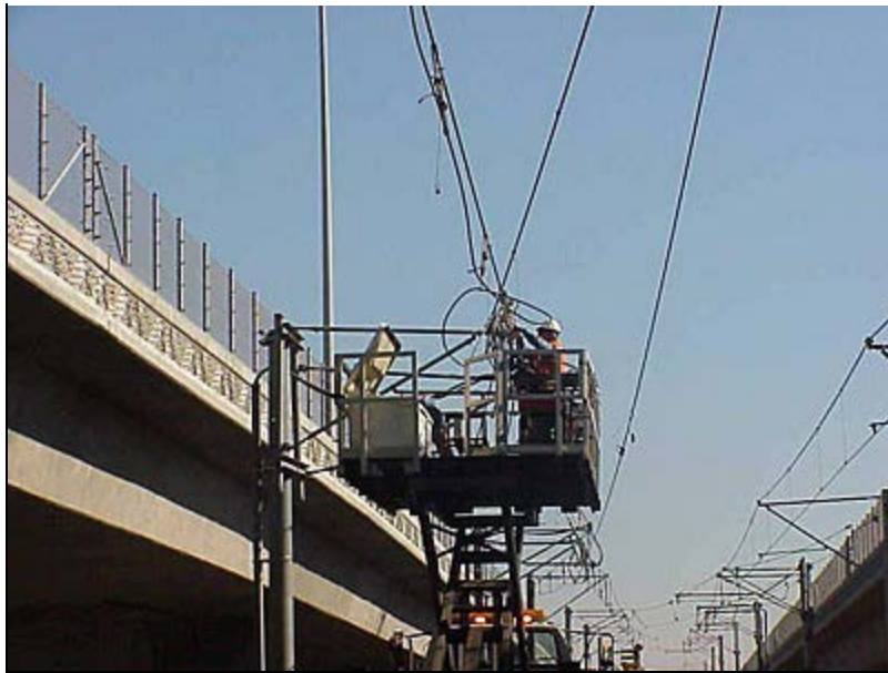
Traction Power Inspectors Tobe Cowden and Frank Hernandez work to repair the downed catenary wire on the Metro Green Line east of the Aviation station.
