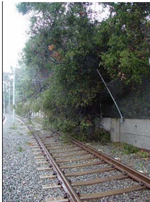
A heavy oak and two smaller eucalyptus trees toppled onto Metro Gold Line power lines in South Pasadena when soggy ground gave way beneath their roots.
