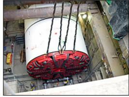
The earth pressure balance machine has cutting edges that grind into the face of the tunnel as the machine inches forward.
