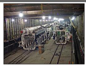
The twin machines are still under construction in this photo. Small rail cars will carry the discharged earth, or muck, away from the rear end of the machines, shown here
