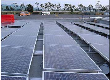
The panels provide 15-20 percent of the two divisions' total energy needs by generating an estimated 700,000 kilowatt-hours per year.
