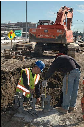
Workers remove bolts which supported temporary signage during construction of the light rail transit bridge.
