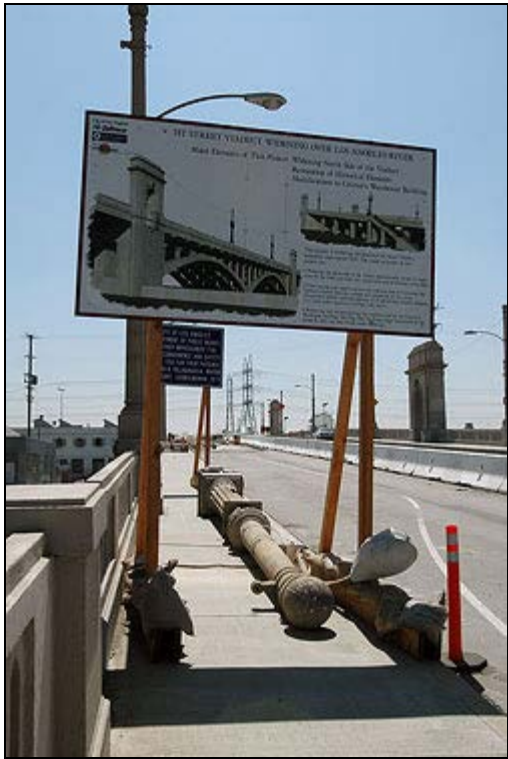
To prepare for arrival of the Metro Gold Line Eastside Extension, the 1 st Street Viaduct across the Los Angeles River is being widened and reinforced. One of the viaduct's historical light standards lies on the sidewalk.
