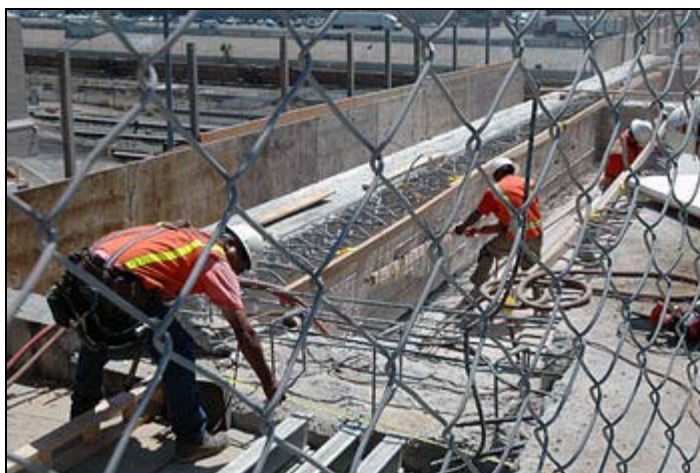
Workers reinforce the girders supporting the 1 st Street Viaduct.
