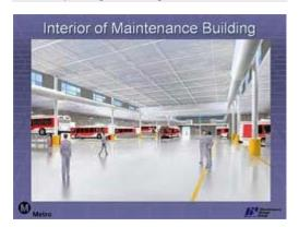
This conceptual view shows a maintenance shop layout that will allow articulated buses to drive straight through with no backing up.
