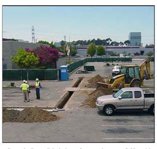
Carson Division 18 is having solar panels installed on new steel shade canopies being placed in its parking lot. This trench will soon be the conduit for power generated by the new panels. The \$4.18 million installation of 1,600 solar panels should pay for itself by 2018. Photo by Jimmy Stroup
