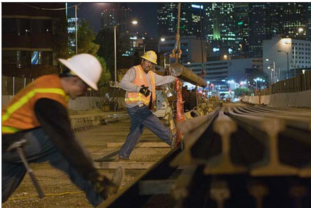
Depending on where intersections fall, the sections being stacked here will be welded together into longer pieces termed "strings."
