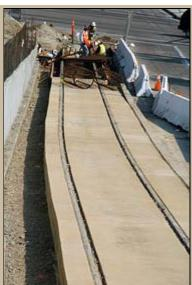
Above, Eastside Extension tracks reach almost to Atlantic Boulevard as workers construct support poles for the overhead power system. The tracks are already installed in the railway.
