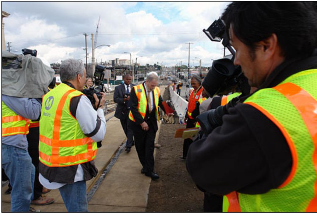
Metro CEO Roger Snoble, sporting one of the newly redesigned reflective safety vests, points out a potentially hazardous footing obstacle to the press and the dignitaries who came to the Eastside Extension construction site, Feb. 20.
