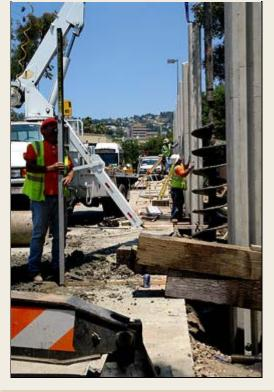
A foreman ensures the columns are being installed correctly by measuring with a laserguided tool. To the right, the massive drill hangs ready to bore the next hole for the next column. Each column is buried 20 feet into the ground to support the 17-foot-high wall. company, Peterson Chase.
