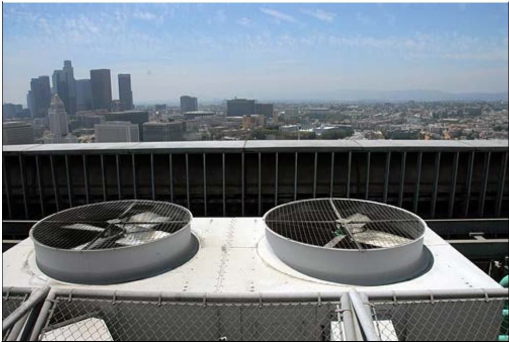
When it gets extremely hot or humid, the massive air conditioning system that cools Metro Headquarters lets off a little steam through the cooling towers on the roof.
