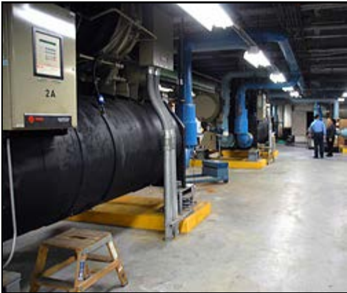
Metro's 1700-ton air conditioning unit includes a configuration of chiller units situated on a floor near the top of the building which funnel water through large pipes that lead to several cooling towers on the roof.
