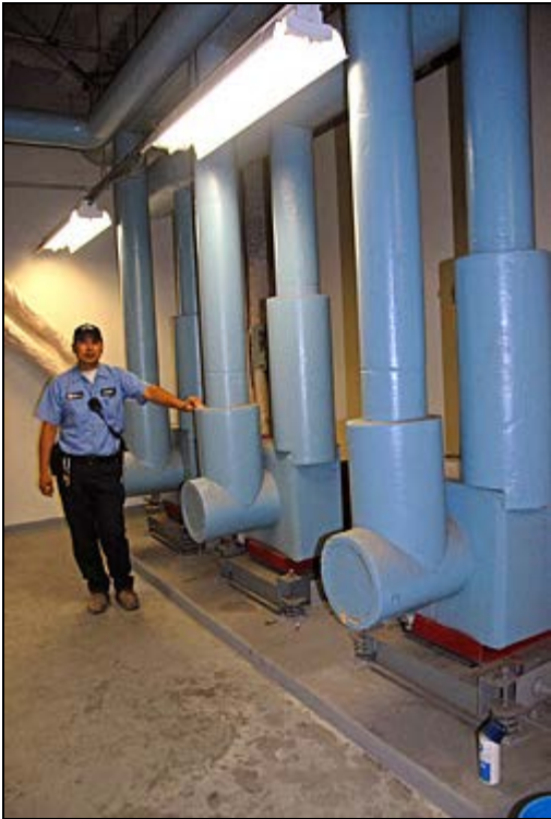
Metro's 1700-ton air conditioning unit includes a configuration of chiller units situated on a floor near the top of the building which funnel water through large pipes that lead to several cooling towers on the roof.
