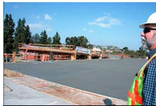
Resident Engineer Matt Gallagher watches as crew lays down last 320 yards of concrete deck to complete top level.
