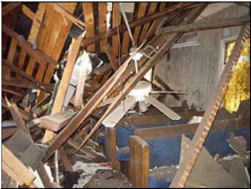
The fallen tree damaged pews, crashed through windows, and left only a rear wall of the church intact.
