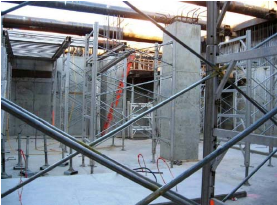
Construction of Boyle Heights Mariachi Plaza Station
