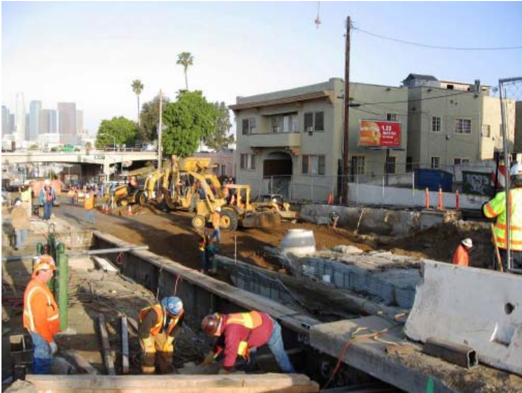
Earth Backfill over the Underground Structures
