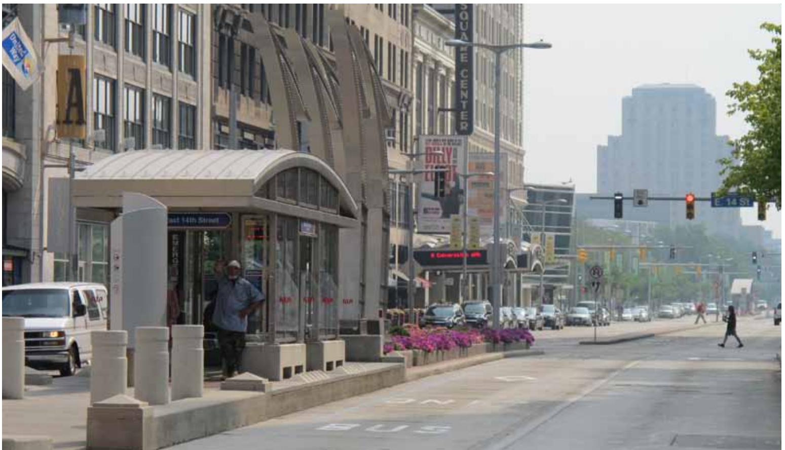
BRT station in Cleveland, Ohio, appropriately set back from the intersection. Photo: ITDP
