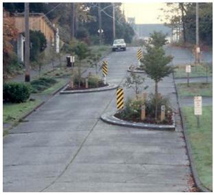
A chicane is used to effectively manage vehicle speeds on a downhill
