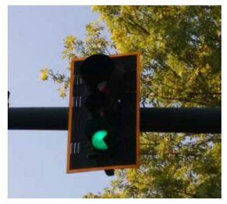
A traffic signal head with Retroreflective border, vented backplate and visors
