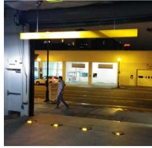
Similar to In-Roadway Warning Lights, beacons are activated when a pedestrian is detected to warn exiting motorists.
