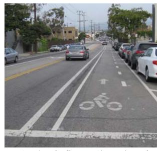
Narrowing a lane of traffic can provide enough room for a buffered bike lane
