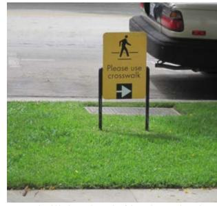
Signage should be located outside of the pedestrian throughway, yet visible from the connecting paths termination point
