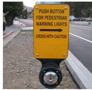
An accessible pushbutton and signage featuring pilot and auditory indicators
