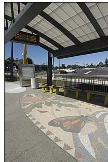
FIGURE 2.8 –Terrazzo Paving at Station
