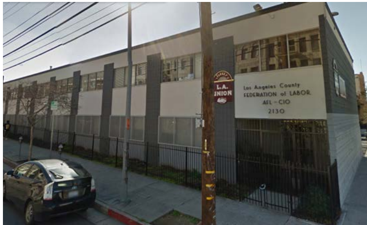
Headquarters of the Los Angeles County Federation of Labor, AFL-CIO (1963), 2130 W. James M. Wood Boulevard (Google Maps)
