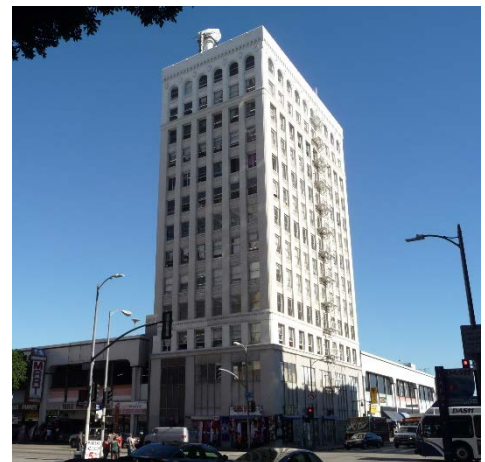
ILGWU (Local 52) Headquarters, per 1929 city directory (1925), 656 S Los Angeles Boulevard (SurveyLA)
