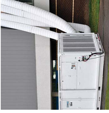
Temporary HVAC system Source: www.esmagazine.com
