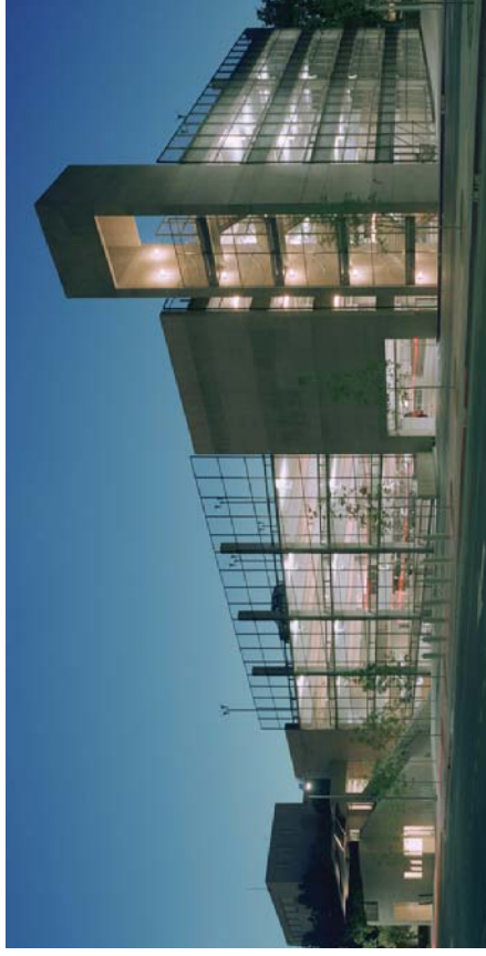
Cornell Parking Structure – Jon Anderson & Antoine Predock – Albuquerque, New Mexico Source: http://jonandersonarchitecture.com
