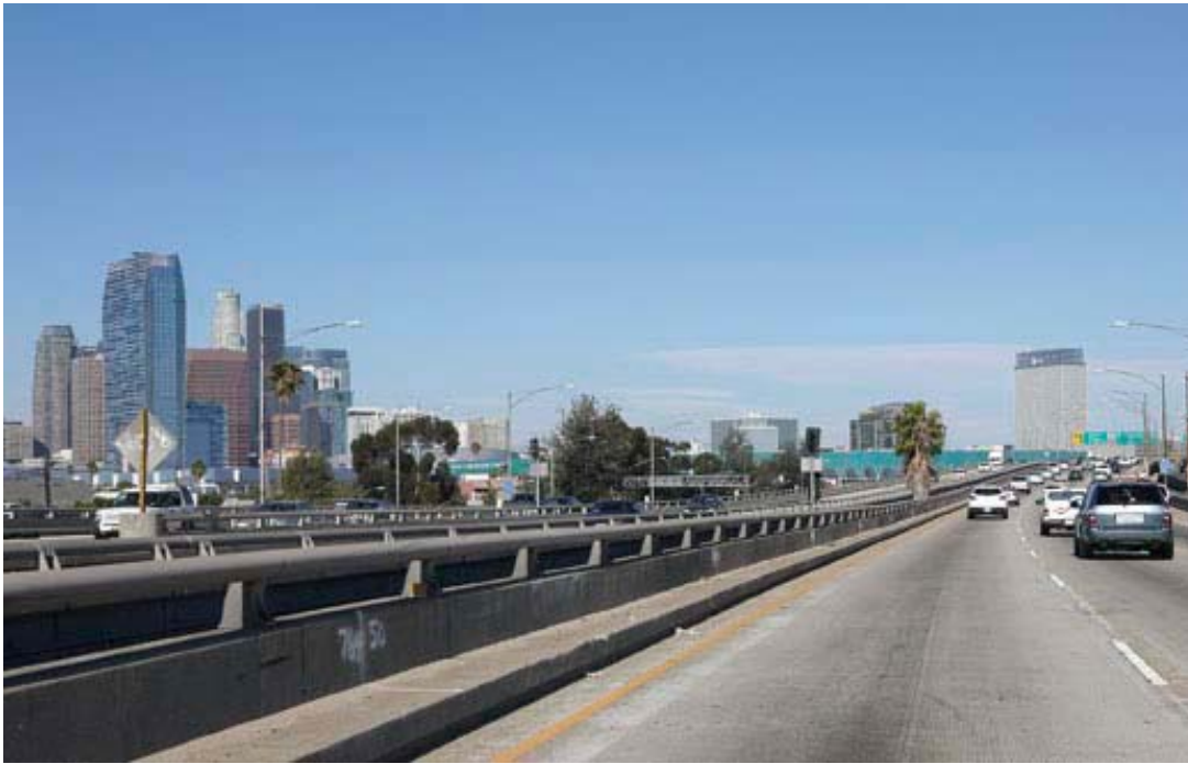
Photo 7a Existing Conditions (Daytime)
