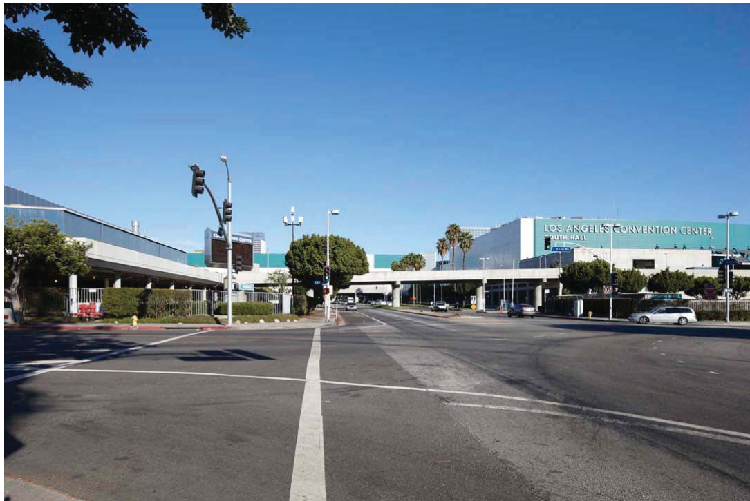
Photo 9a Existing Conditions (Daytime)
