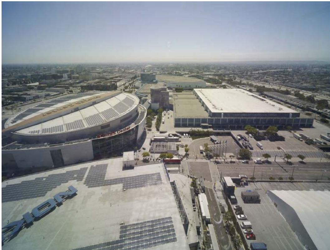
Photo 15a Existing Conditions (Daytime)
