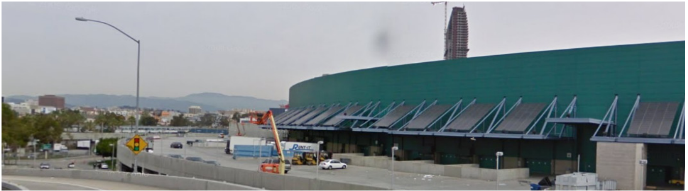
Figure 3.3.3.3 - Photograph of daytime view from Receptor 5. (Photo courtesy Google: google.maps.com)
