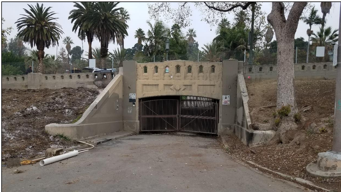
Figure 11. View of the Wilshire Boulevard underpass.
