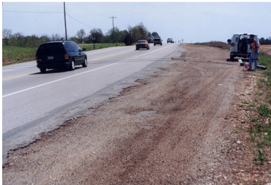
FIG. 3-1 US 65 SB Station 1
