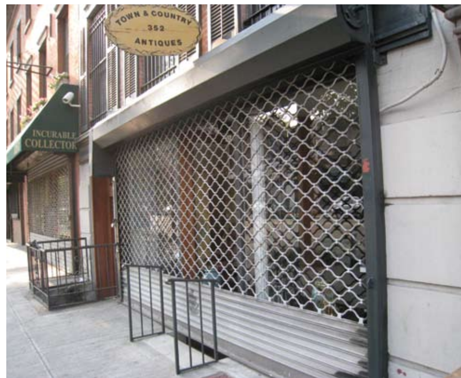
Open-grilled gates maintain safety but create a more interesting building front along the sidewalk.
