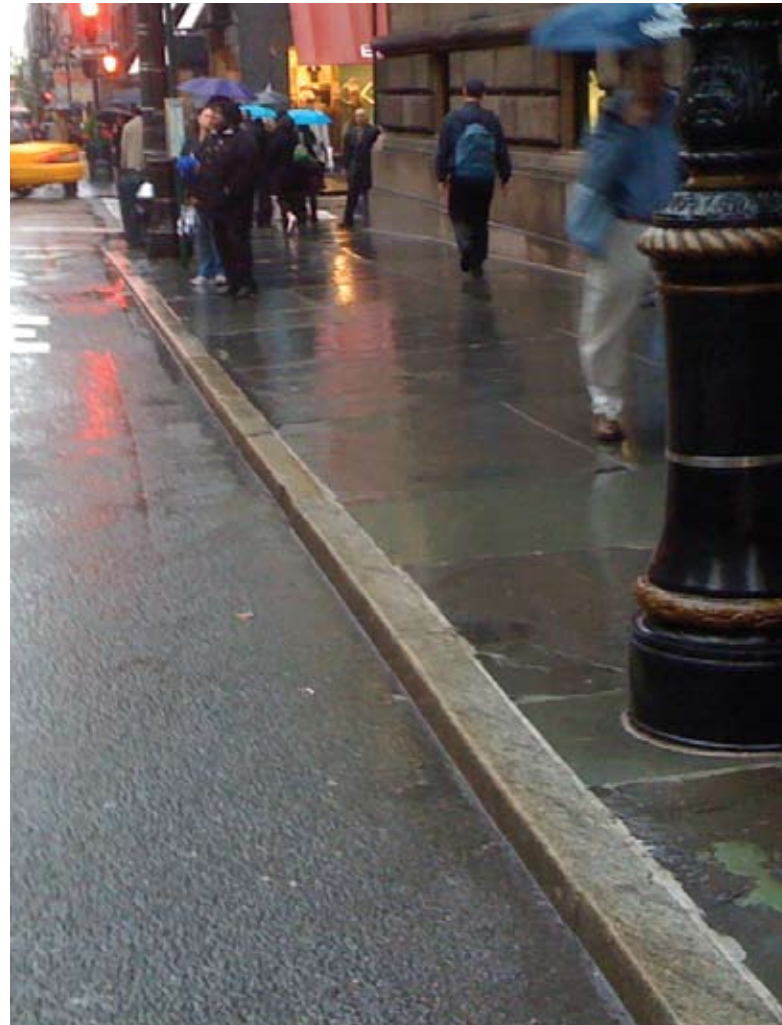
Granite saw-finished curb, Madison Avenue, Manhattan.
