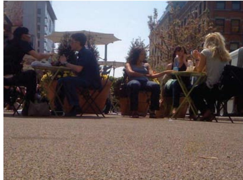
Resin-bound gravel, 9th Avenue & 14th Street, Manhattan.
