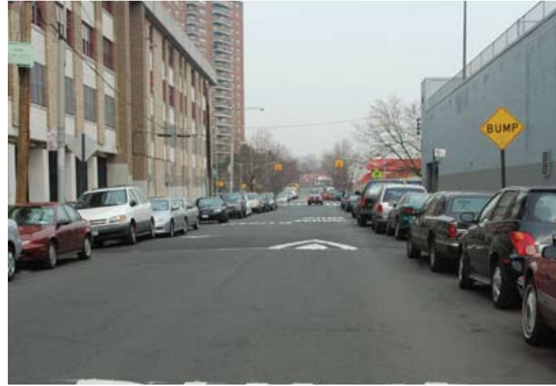
Raised speed reducers, Bolton Avenue, Bronx.
