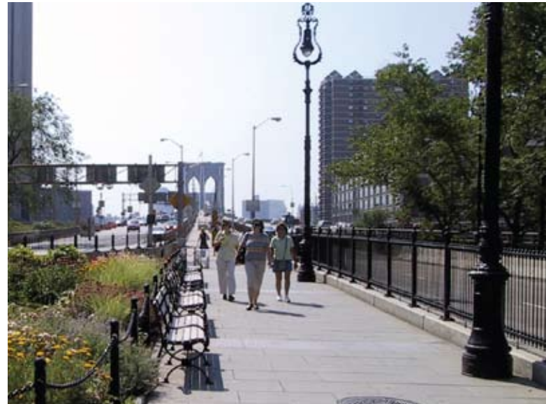
London pavers, Brooklyn Bridge pedestrian ramp.
