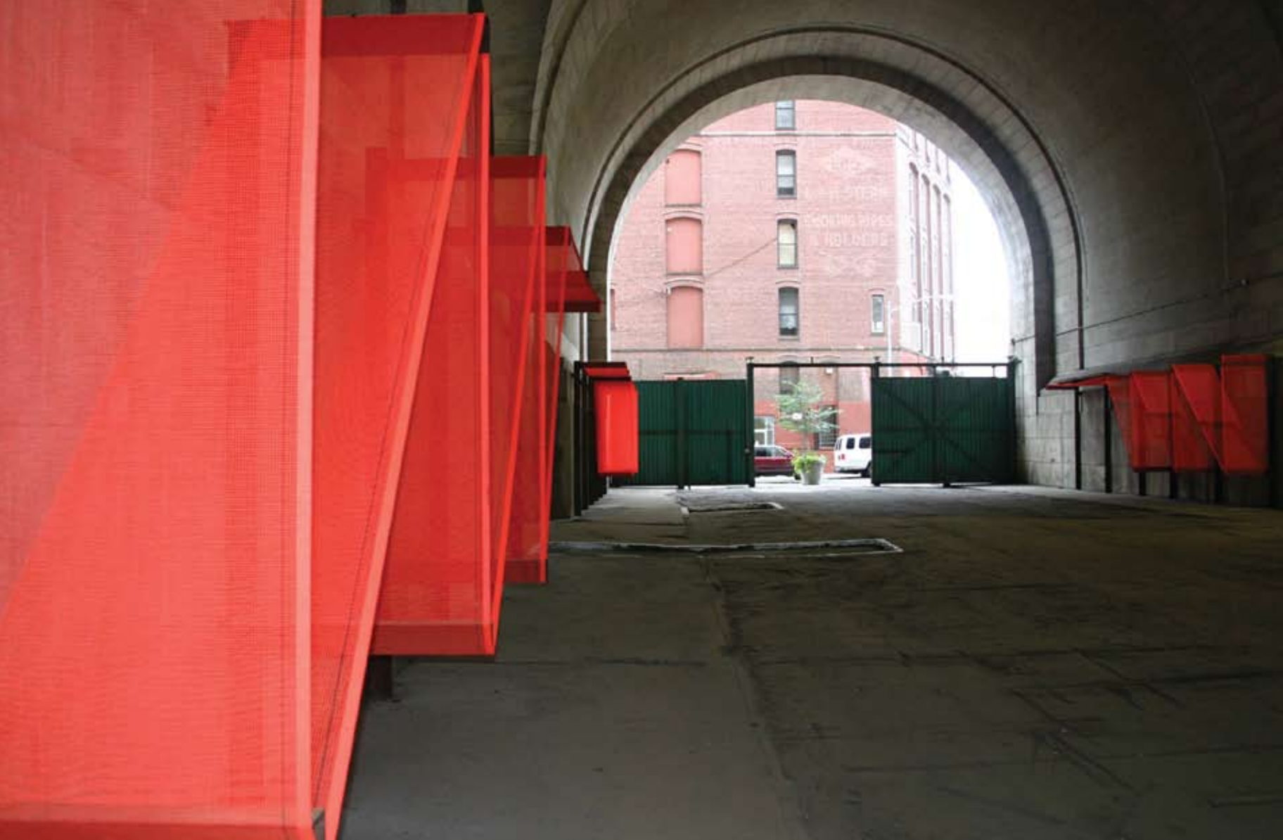
Manhattan Bridge Arch, Brooklyn.
