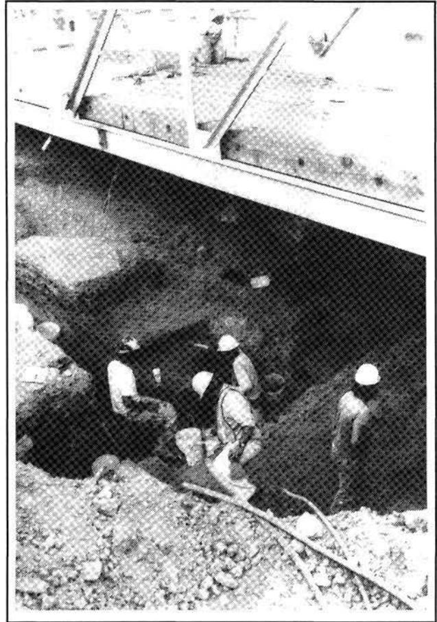
Figure 1.4. Excavation Under the Passenger Bridge (Locus 1)
