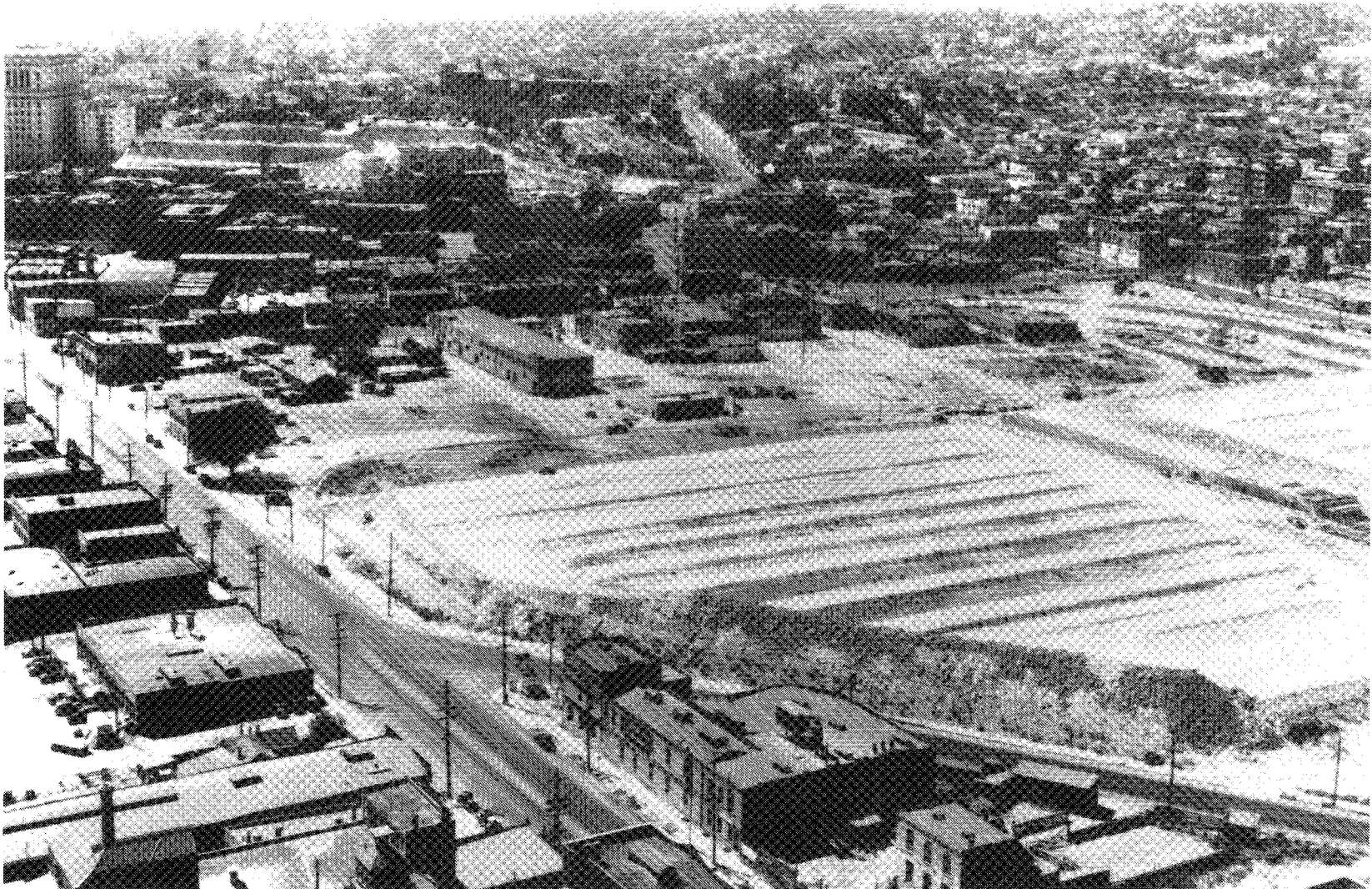
Figure 9.4. Project Area after Demolition and Filling
