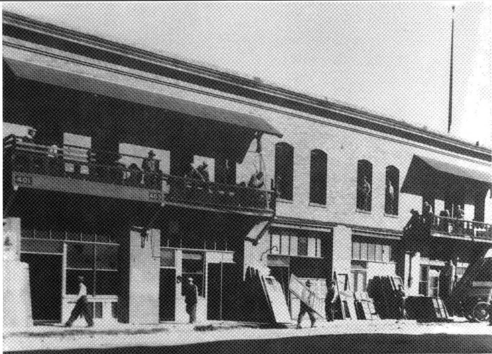
Figure 2.14. Demolition Begins at 401-403 Apablasa Street (Courtesy, Collection of Carlos Apablasa)
