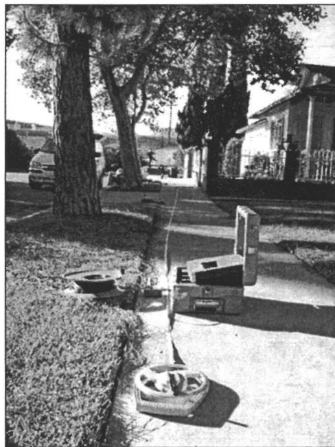
Figure A-14. Site V-4, End of Caroline Avenue, North of National Boulevard
