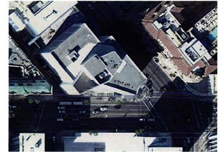
Entrance 2, Aerial View
