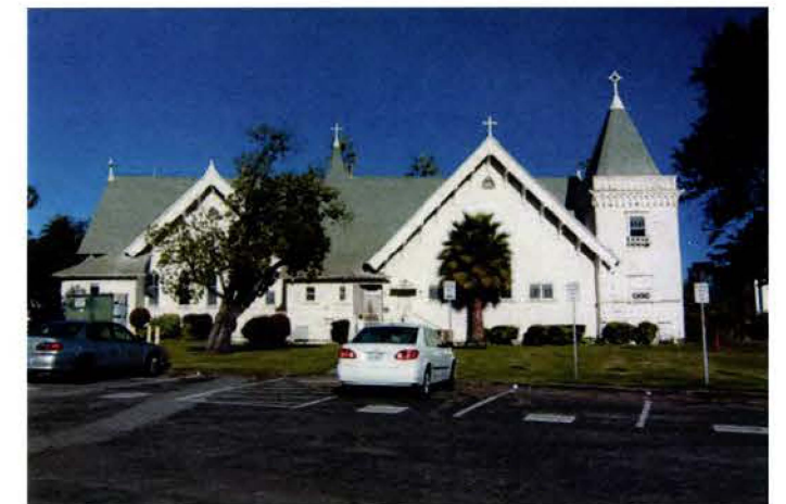
Photo of historic Wadsworth Chapel near VA north station option
