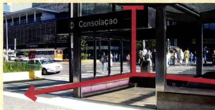
Consolação Station: São Paulo, Brazil. Queuing area does not affect station entrance with perpendicular entrance.
