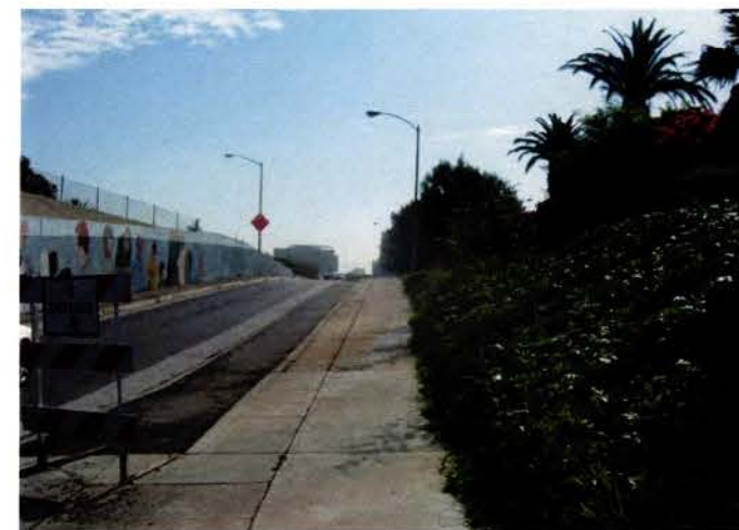
View of existing slip road headed east that will be realigned to the south to separate the station plaza from the VA hospital area.
