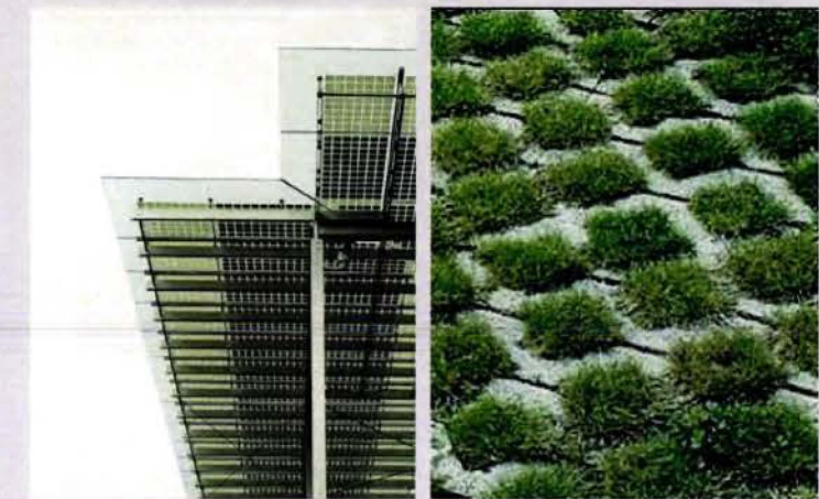
Solar panel roof generates energy and provides shade.
