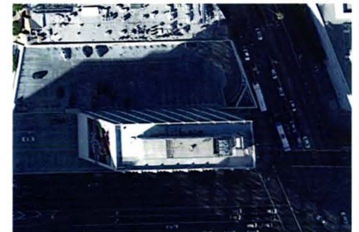
Entrance 2, Aerial View
