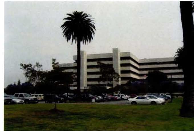
Entrance 1, looking south
