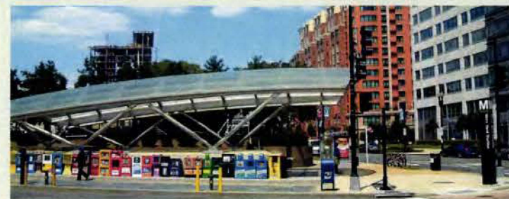
Station portal in Navy Yard Area in Washington, D.C. is oriented toward the main street and intersection for easy pedestrian orientation.
