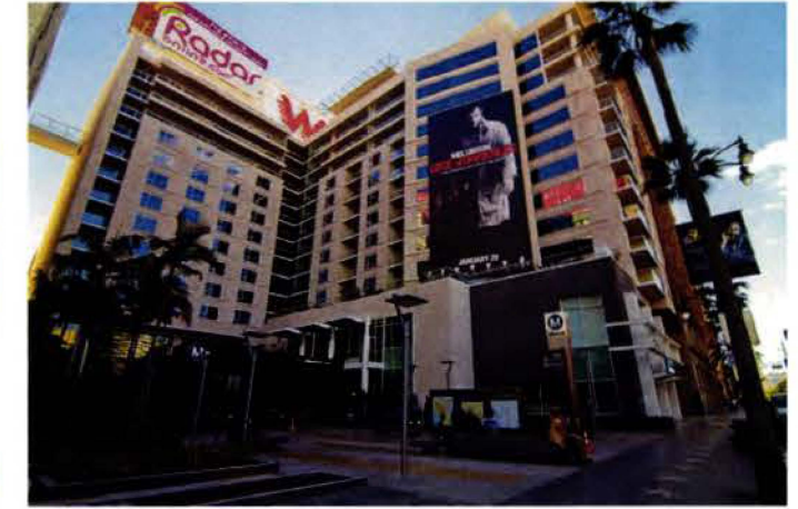
Photo of recent joint development at Hollywood/Vine station
