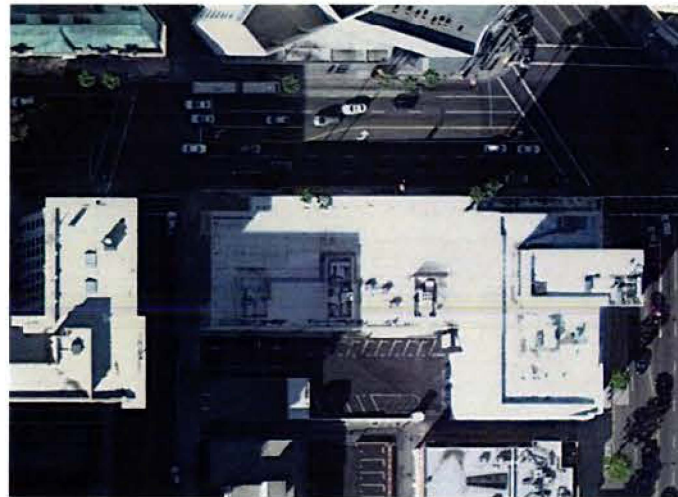
Entrance 1, Aerial View
