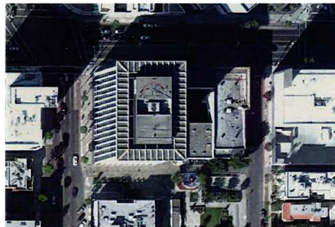
Entrance 3, Aerial View
