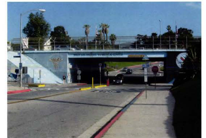
View of Wilshire bridge, looking south from VA north station option
