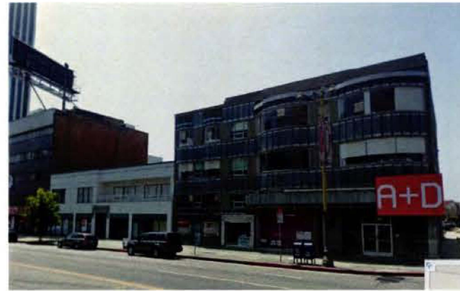
Entrance 3, looking south toward A+D museum
