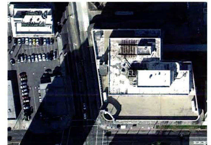
Entrance 2, Aerial View
