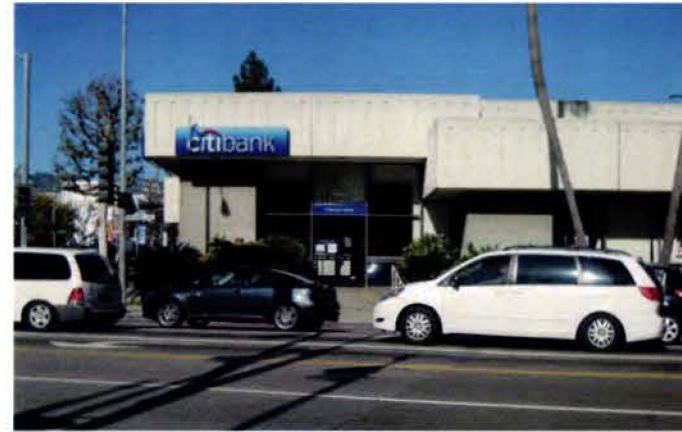
Entrance 1, looking north toward Citibank parcel
