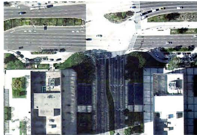
Entrance 3, Aerial View
