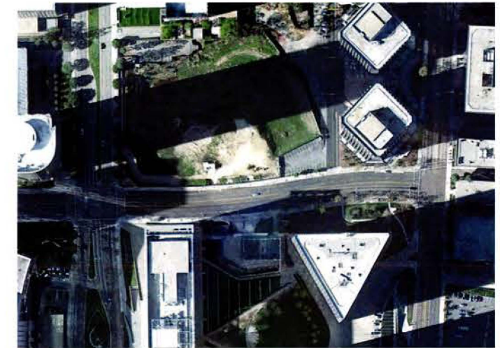
Entrance 2, Aerial View
