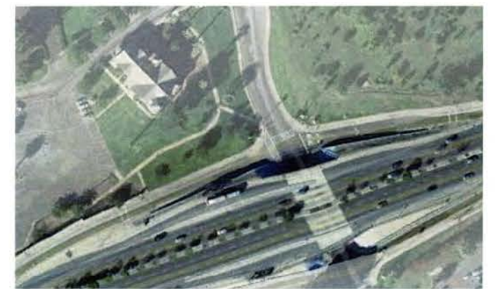
Entrance 2, Aerial View
