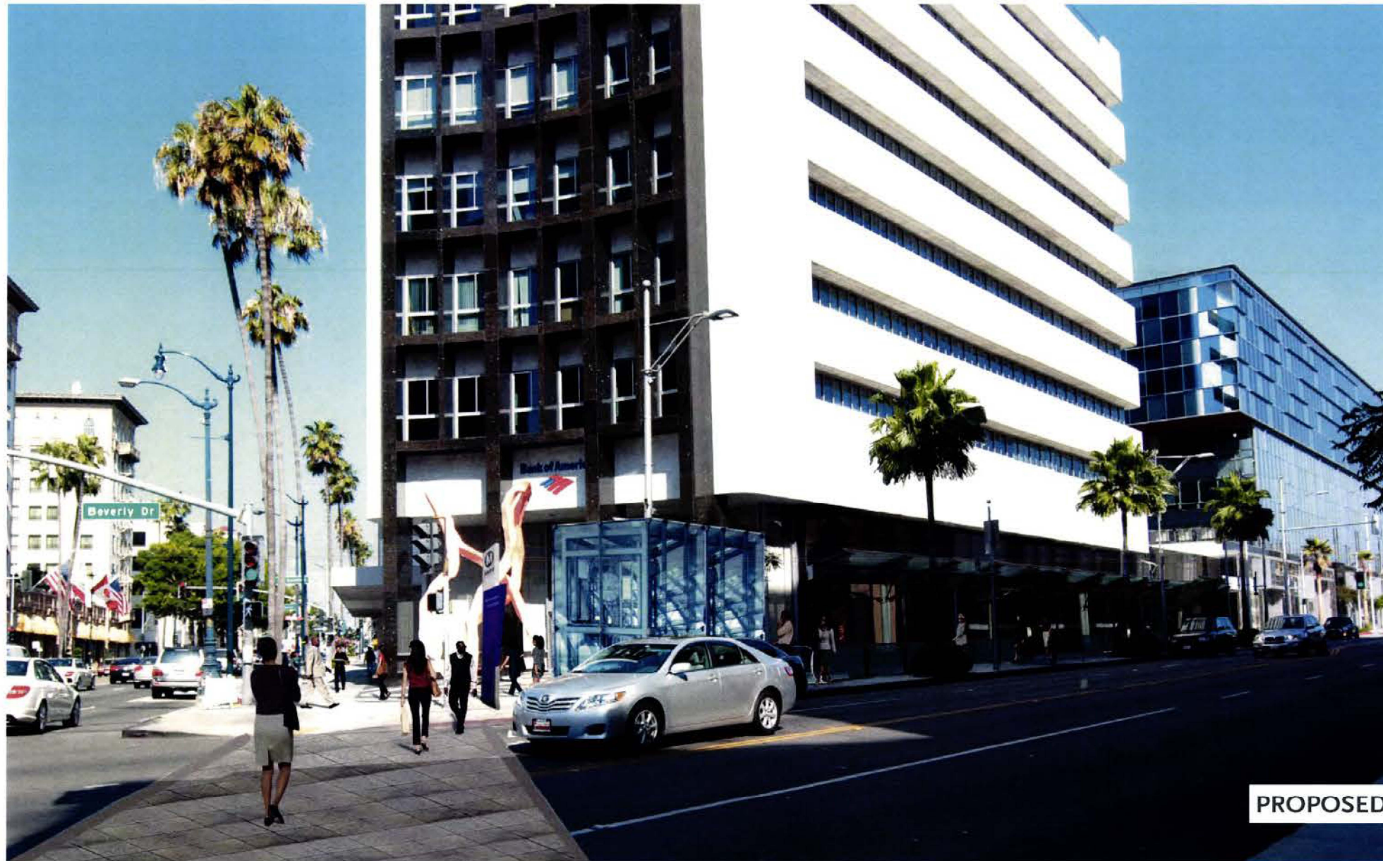
"After" photo montage of Bank of America West entrance, looking west down Wilshire.
