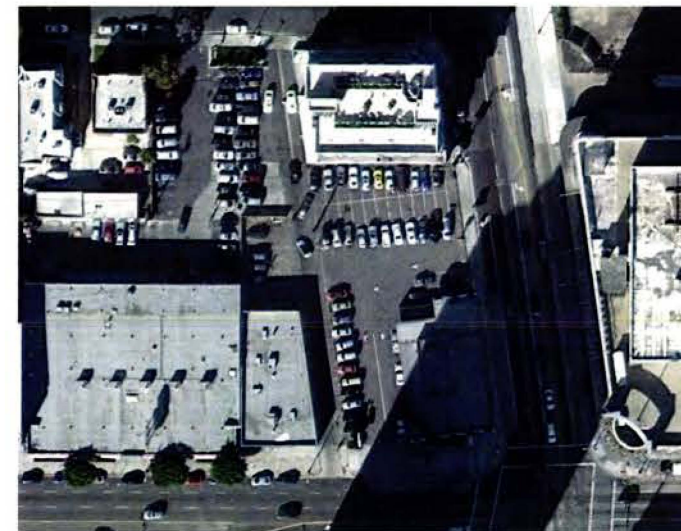
Entrance 1, Aerial View
