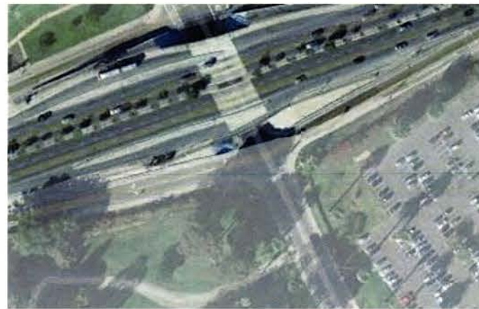
Entrance 1, Aerial View
