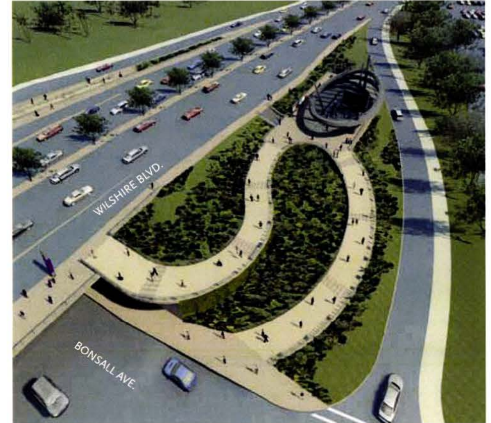
View of station area with ramps coming down from Wilshire bus drop off area to station plaza along Bonsall. The on-ramp from Bonsall to Wilshire is realigned to the south to separate the VA Hospital from the Metro station operations.
