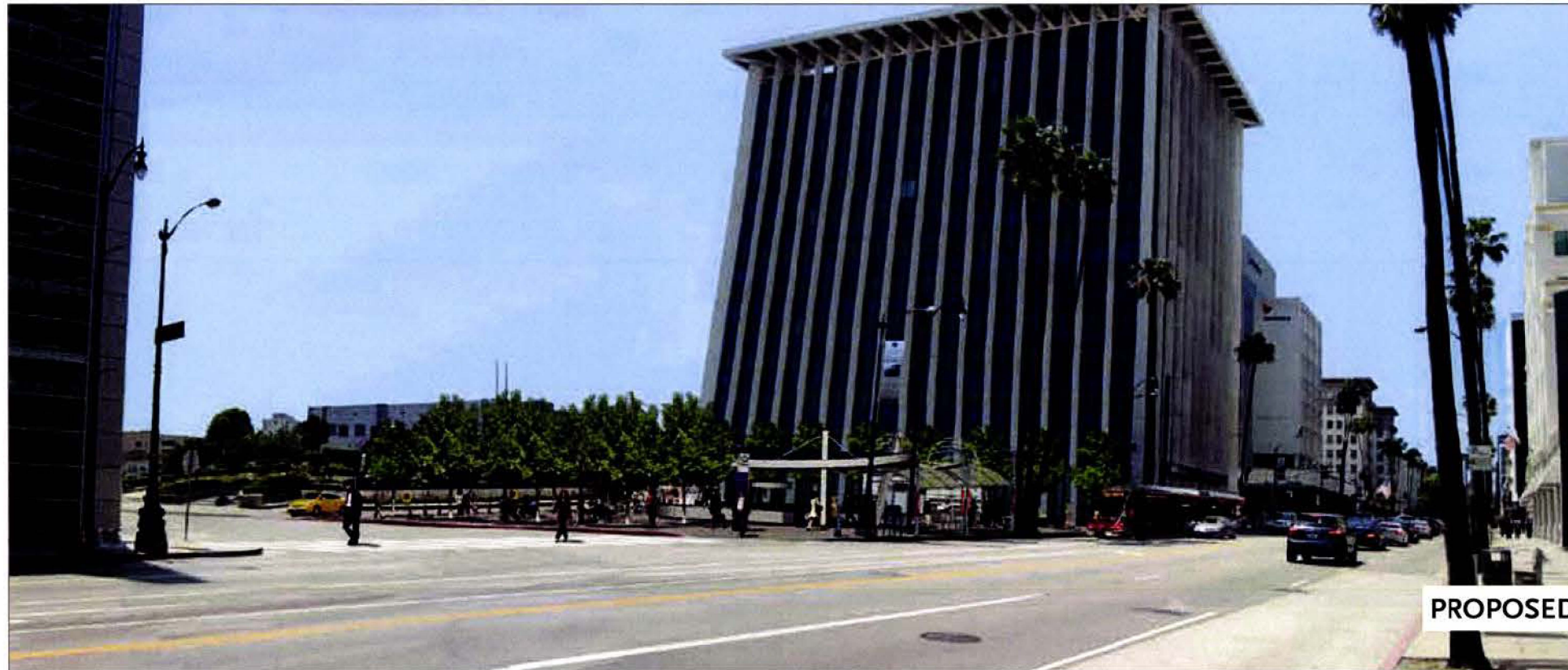
"After" photo montage of ACE Gallery entrance with plaza providing a grove of trees, seating, and taxi drop off and pick up along the alley behind the parcel.
