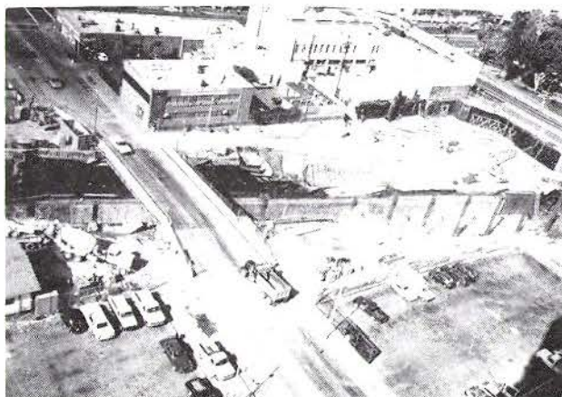
OVERHEAD VIEW OF STATION CONSTRUCTION PROGRESS. WESTLAKE AVE WESTWARD
