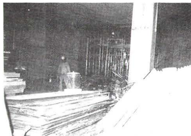
REMOVING SUPPORTS AFTER POURING OF ROOF SLAB IN THE NORTH BLAST RELIEF SHAFT
