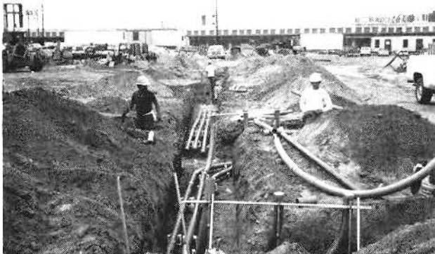
INSTALLATION OF NEGATIVE RETURN DUCT BANKS, NORTH OF THE MAIN SHOP BLDG.
