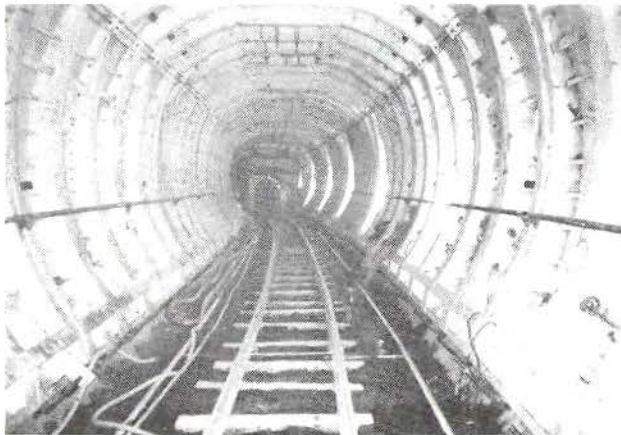
ARCH FORMS IN PLACE AL TUNNEL
