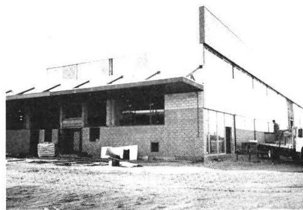
NORTHWEST CORNER OF BUILDING. FIRST FLOOR FRONT AND SECOND FLOOR WINDOWS ARE INSTALLED
