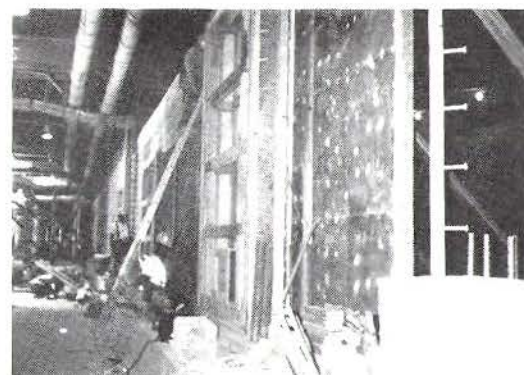
LRT INTERIOR WALLS
