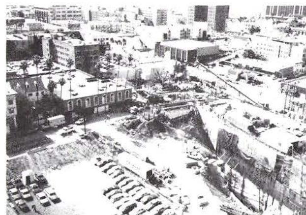
OVERHEAD VIEW OF STATION CONSTRUCTION PROGRESS AT EAST END OF STATION A171/A175 INTERFACE
