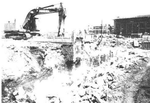
DEMOLITION OF EXISTING LAUPT UTILITY TUNNEL AND PASSENGER TUNNEL RAMP
