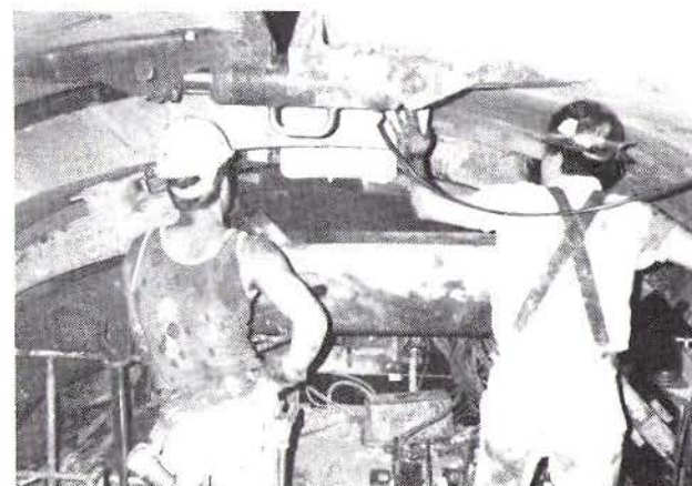
WORKMEN USING HYDRAULIC ERECTOR TO INSTALL PRECAST CONCRETE TUNNEL SEGMENTS
