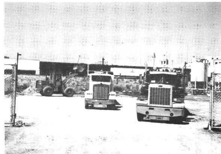
LOADING OF HYDROCARBON CONTAMINATED SOIL TEMPORARILY STOCK PILED AT A144 SITE FOR HAULING TO PECK ROAD DISPOSAL FACILITY
