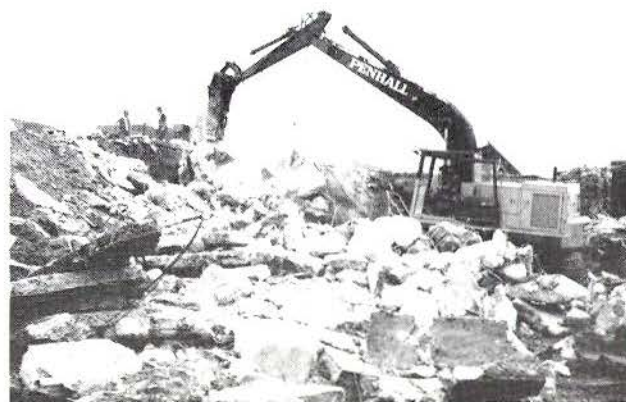
DEMOLITION OF UTILITY TUNNEL, PASSENGER RAMPS AND PLATFORMS WITHIN LAUPT TRACKYARD
