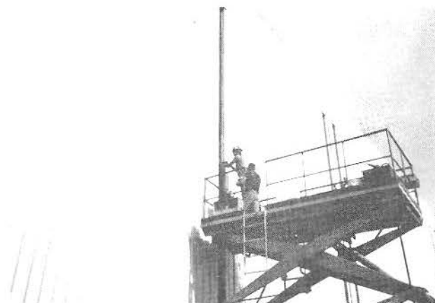
COLUMN COVER BEING INSTALLED ON "B" LINE
