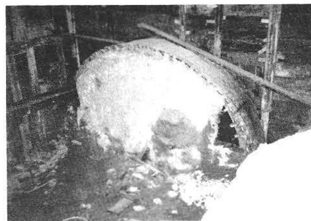
A165/A171 INTERFACE WITH A171'S SHIELD AND THE CONCRETE BULKHEAD INSIDE THE A165 STATION LIMITS
