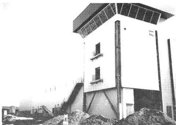
CONTROL TOWER - SUBSTANTIALLY COMPLETE
