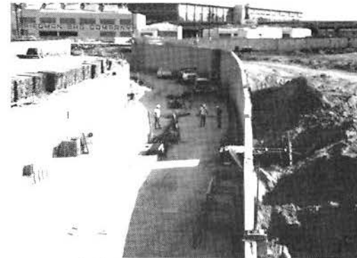
"U" WALL STRUCTURE - RETAINING WALLS COMPLETE
