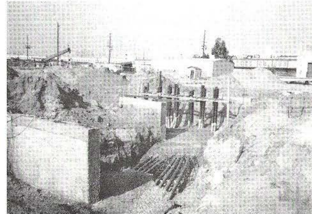
DUCT BANKS LEADING TO OPERATING PLATFORM NO. 3, LOOKING SOUTHWEST TOWARDS SANTA FE AVENUE
