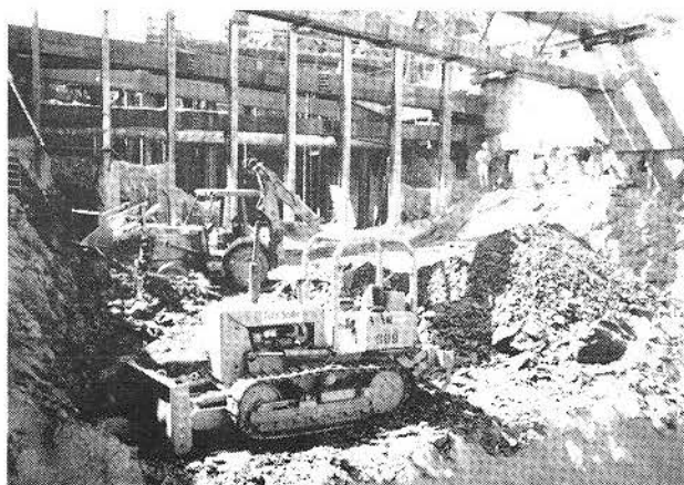
EXCAVATION AND SUPPORT OF EXCAVATION AT A171/A175 INTERFACE
