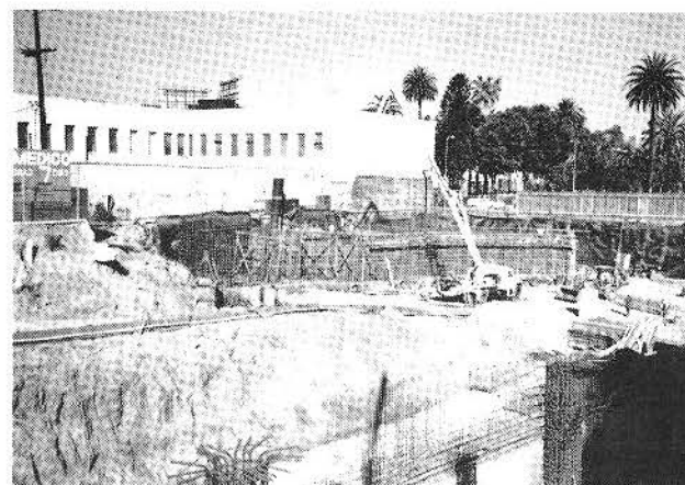
PLACEMENT OF WALLS FOR THE SOUTH INTAKE AND EXHAUST SHAFTS
