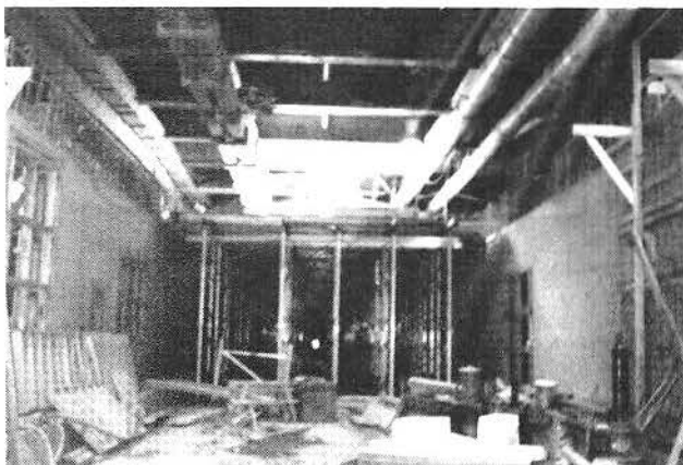
LRT INTERIOR WALLS
