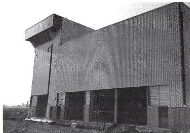
NORTHSIDE OF BUILDING SHOWING CONTROL TOWER AND S & I PIT ENTRANCES
