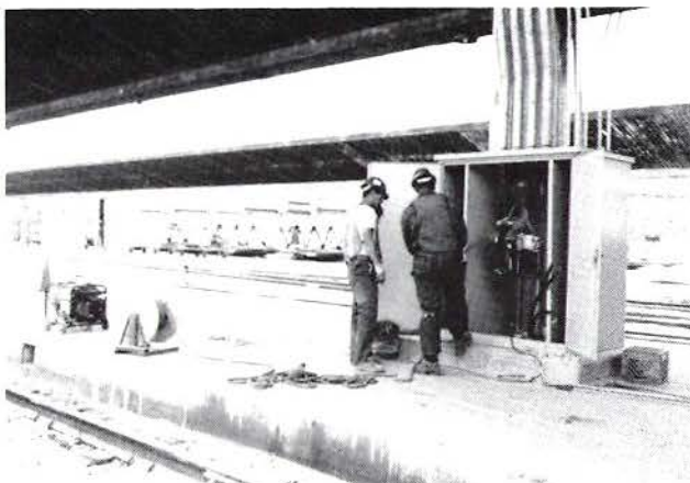
INSTALLATION OF CABLE IN NEW PULL BOX #7 WITHIN LAUPT TRACKYARD
