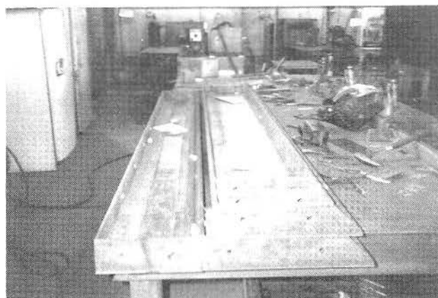
WALKWAY FORM UNDER FABRICATION IN STEEL SHOP
