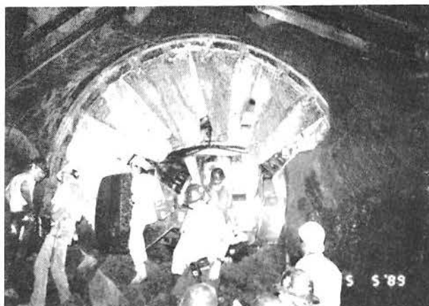
BREAK THRU OF AR TUNNEL INTO NORTH END OF CIVIC CENTER STATION
