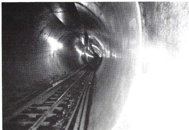
AL TUNNEL ARCH LOOKING EAST AT STA. 242+50
