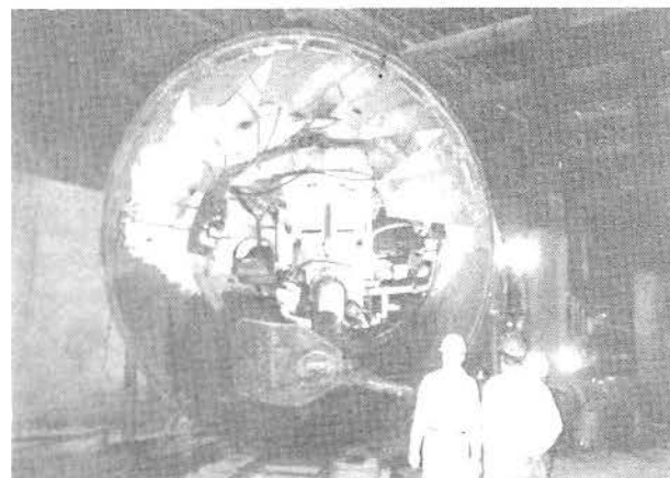
MOVING TUNNELING MACHINE THROUGH S CURVE TO AL TUNNEL AT SOUTH END OF CIVIC CENTER STATION
