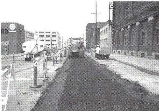
PERMANENT PAVEMENT RESTORATION AT 3RD STREET IN CONNECTION WITH SEWER LINE WORK, LOOKING WEST FROM SANTA FE AVENUE
