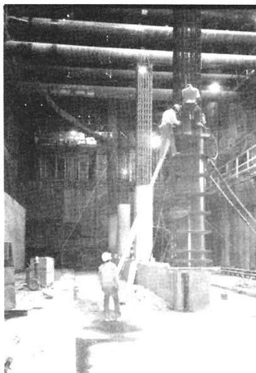
POURING CONCRETE COLUMN IN CIVIC CENTER STATION
