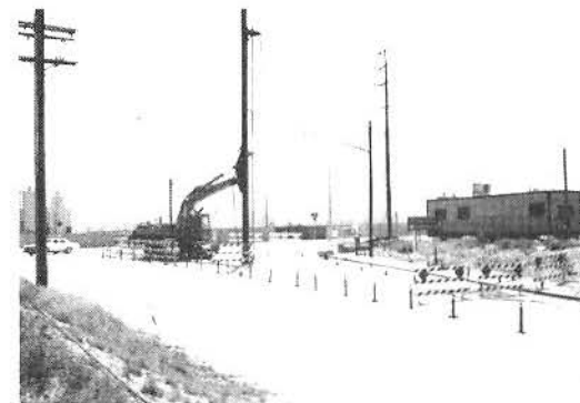
DRILLING HOLES FOR CHEMICAL GROUT STABILIZATION
