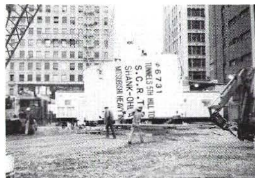
PART OF SHIELD FOR AR TUNNEL BEING LOWERED ONTO BLOCKS
