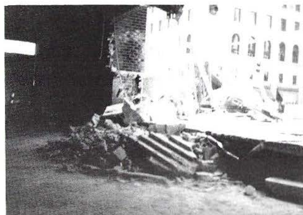
DEMOLITION AT ROOSEVELT BUILDING (OLD REPUBLIC BANK)
