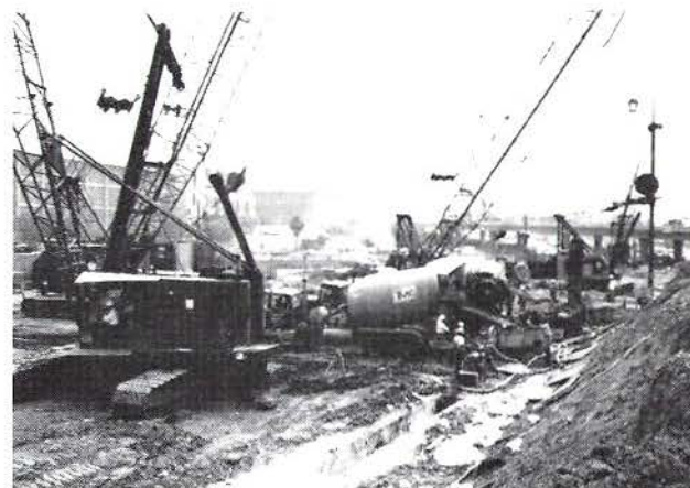
PLACING CONCRETE FOR SLURRY WALL PANEL IN PHASE I STAGE I SECTION
