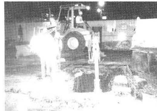
SANITARY SEWER MANHOLE C-1 INSTALLATION IN 4TH STREET
