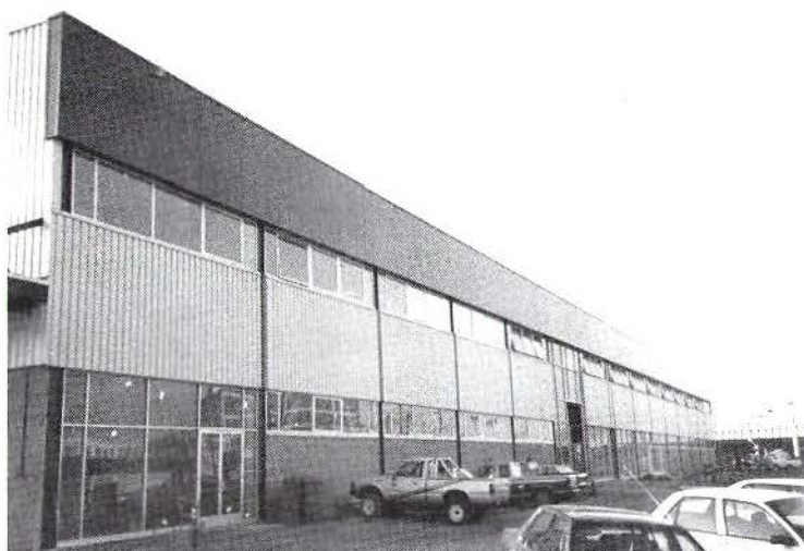
FRONT VIEW OF MAIN SHOP BUILDING (WEST SIDE) SHOWING MAIN ENTRANCE
