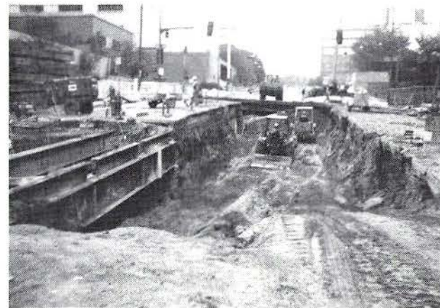
BACKFILLING HILL STREET SOUTH OF FIRST ST. OVER THE SOUTH BLAST RELIEF SHAFT
