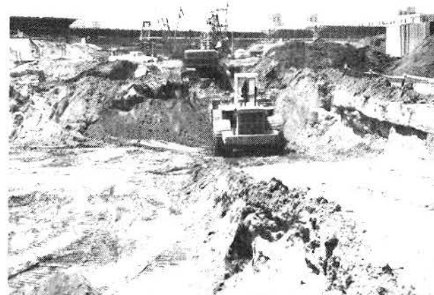
STRUCTURE EXCAVATION IN SLURRY WALL AREA
