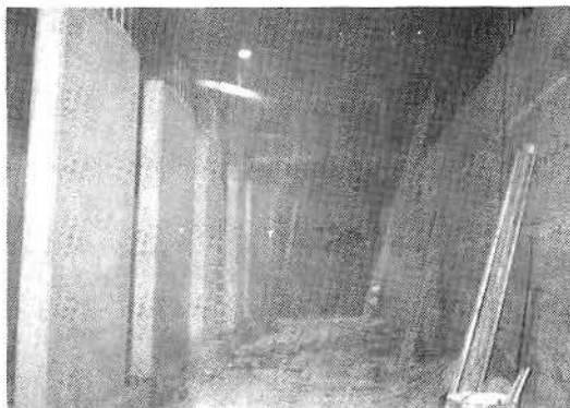
LRT CENTRAL WALLS AT NORTH BULKHEAD ON FLOWER STREET
