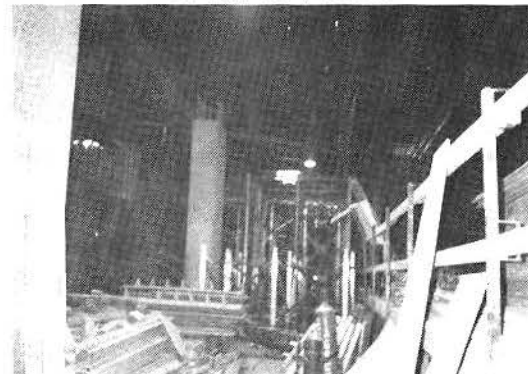
LRT INTERIOR COLUMNS, SOUTH OF 7TH ST. ON FLOWER ST.
