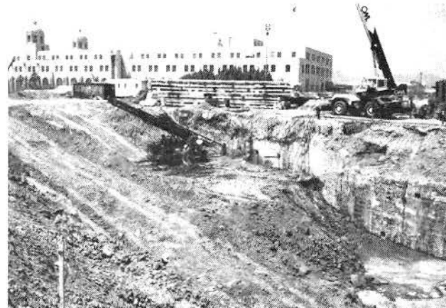
DRILLING OPERATION FOR SLURRY WALL TIEBACKS
