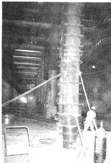
PREPARING TO POUR COLUMN CONCRETE AT CIVIC CENTER STATION
