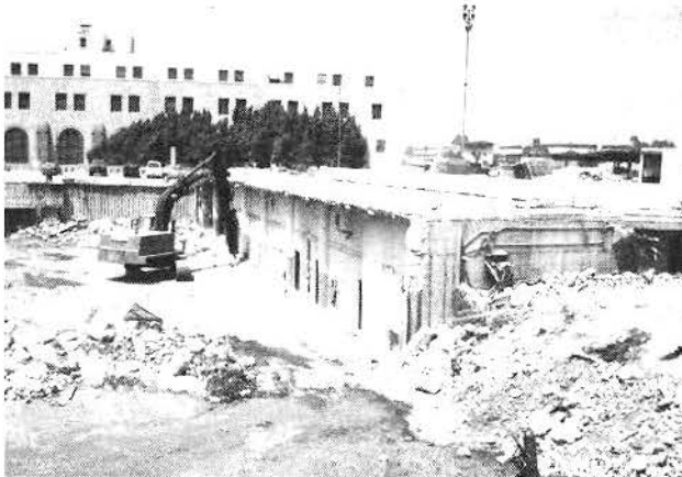
DEMOLITION OF STREET LEVEL SLAB OF THE REA BUILDING
