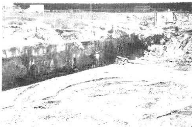
EXPOSED SLURRY WALLS
