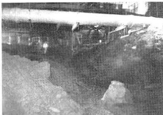
TEMPORARY SANITARY SEWER LINE-C, SUPPORTED AT THE NORTH END OF STATION, UNDER 4TH STREET
