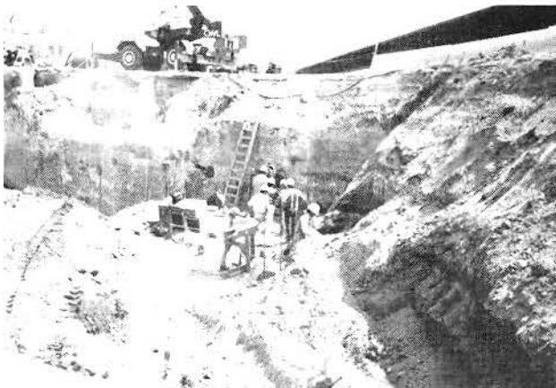
BACKGROUND: SLURRY WALL TIEBACK ANCHOR TESTING FOREGROUND: ARCHEOLOGICAL EXCAVATION
