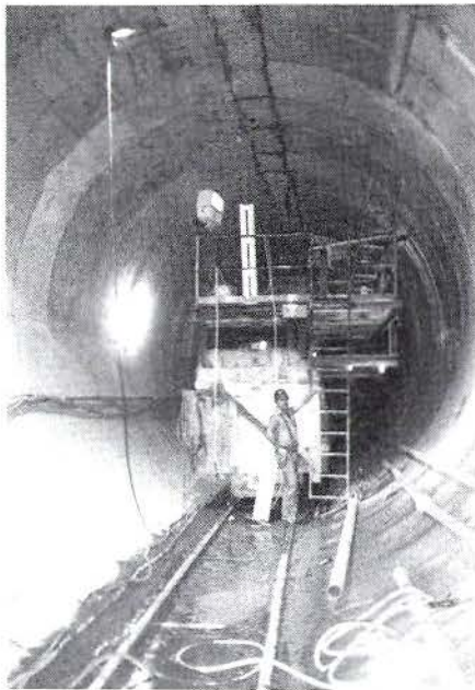
PLATFORM MOUNTED ON RAILCAR FOR SAWCUTTING CONCRETE SEGMENTS PRIOR TO CROSS PASSAGE EXCAVATION IN AL TUNNEL
