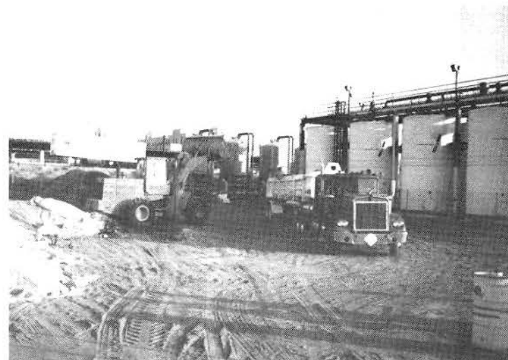
CONTAMINATED SOIL BEING LOADED FROM TEMPORARY STORAGE FACILITY PRIOR TO DISPOSAL
