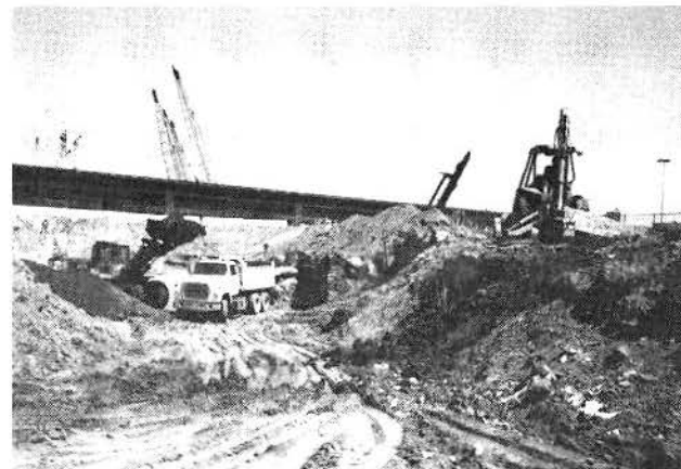
EXCAVATION TO ELEVATION 272 IN WEST AREA OF TRACK YARD
