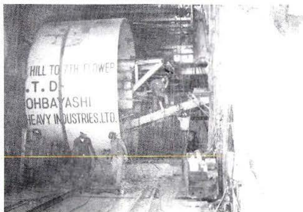
SHIELD JACKED FORWARD BY 9 FEET INTO AR TUNNEL; MUCK REMOVAL CONVEYOR BEING ASSEMBLED
