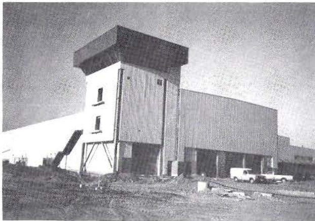
CONTROL TOWER, BLOWDOWN FACILITY AND NORTH ENTRY TO S & I AREA
