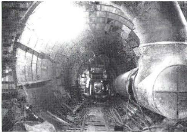
AL TUNNEL LOOKING SOUTH FROM CIVIC CENTER STATION
