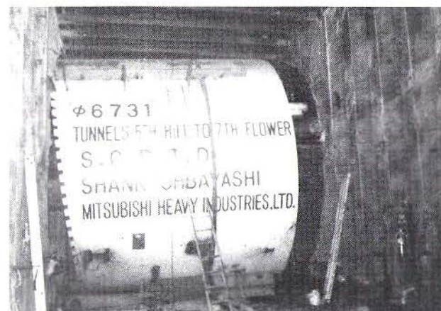
SHIELD IN POSITION AT PORTAL OF AR TUNNEL; CONCRETE SADDLE BEING POURED BENEATH SHIELD
