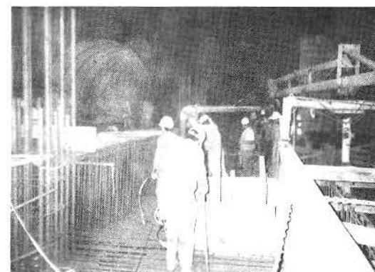
POURING CONCRETE FOR INVERT #1 AT NORTH END OF CIVIC CENTER STATION
