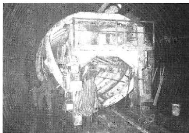
FORM CARRIER MOVING ARCH FORMS IN AR TUNNEL
