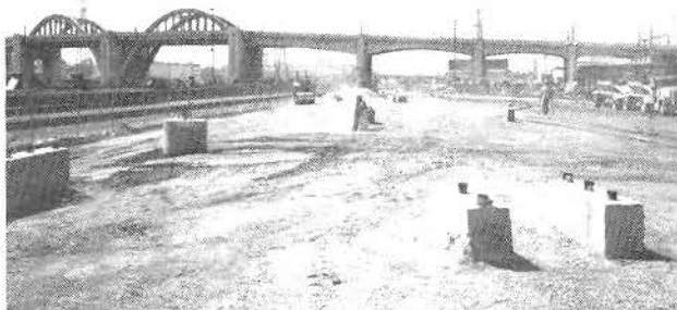
STARTED PLACEMENT OF INITIAL BALLAST FOR TAIL TRACKS, LOOKING SOUTH TOWARDS 6TH STREET BRIDGE
