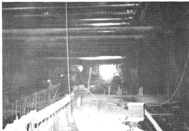
MRT BASE SLAB WEST OF FLOWER ST. ON 7TH ST. A171 TUNNELS IN THE BACKGROUND
