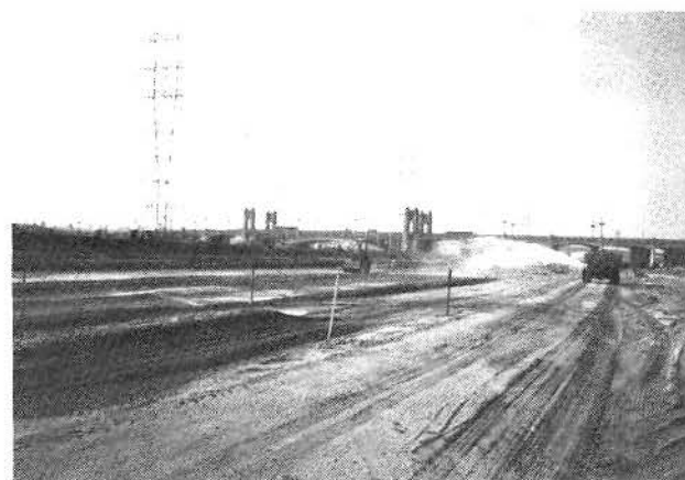
CONTINUED PLACEMENT OF SUBBALLAST, BASE LINE STATION 23+00 TO 27+00, TRACKS 1 THRU 9, LOOKING SOUTH TOWARDS 4TH STREET BRIDGE
