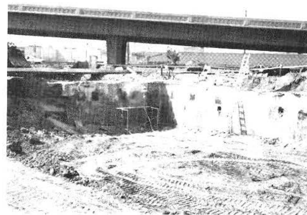
EXPOSED SLURRY WALLS
