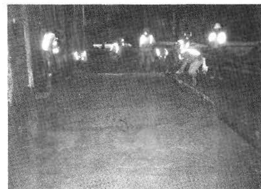
POURING THE 4-INCH MUD-MAT AT THE STATION'S SOUTH END, INVERT 16/15
