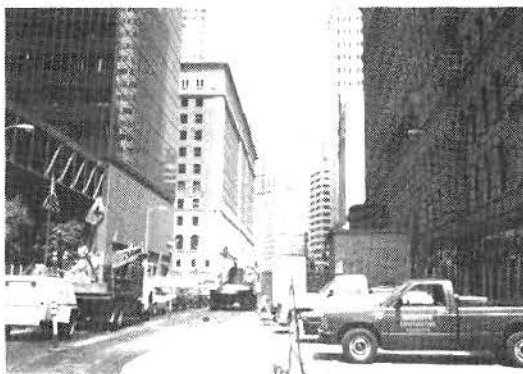
CONSTRUCTION LAYDOWN AREA, ON NORTH SIDE OF 7TH ST. EAST OF FLOWER ST.
