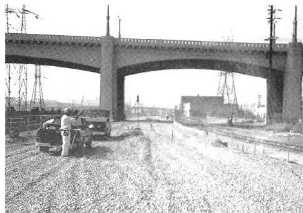
GRADING INITIAL BALLAST AT 6TH ST. AREA
