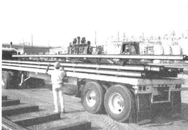
UNLOADING AND STORING CONTACT RAILS AT YARD SITE
