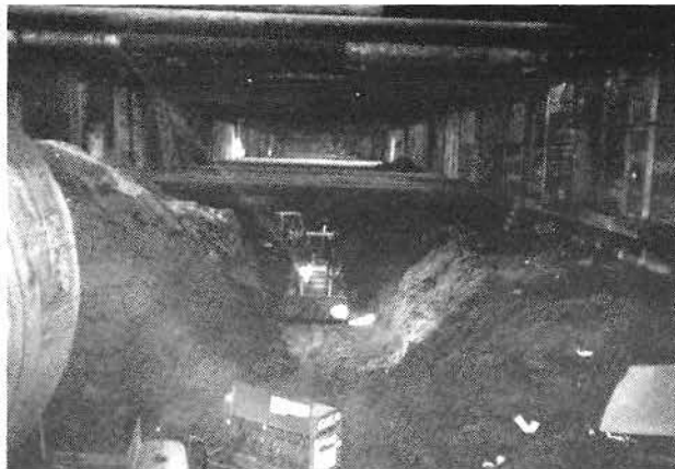
OVERVIEW OF THE STATION'S EXCAVATION NORTH TO SOUTH. SHOWN ARE LEVEL 3 AND 4 STRUTS AND BORING MACHINE (PART OF) TO THE LEFT
