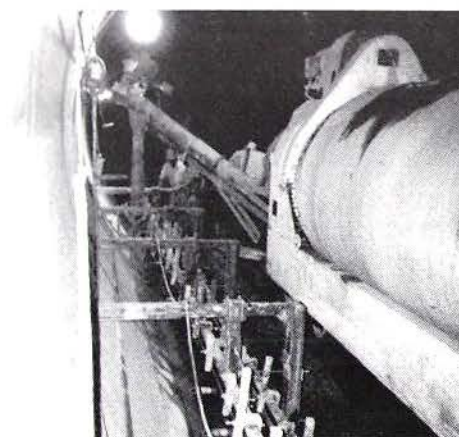
MORAN CONCRETE CAR IN PLACE FOR WALKWAY CONCRETE
