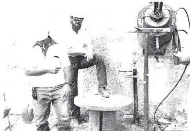
STRESSING TIEBACKS IN SLURRY WALL
