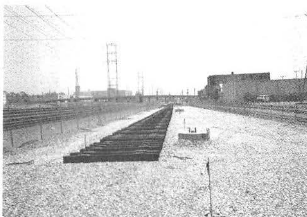
PLACING TIES FROM SOUTH OF 6TH ST. TO SOUTH END OF PROJECT
