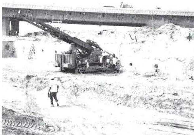
DRILLING FOR SLURRY WALL TIEBACKS
