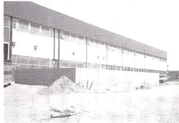
LUNCH PATIO RETAINING WALL. TRELLIS SUPPORTS ON COLUMNS. EXTERIOR LIGHTS PARTLY INSTALLED ON FACADE
