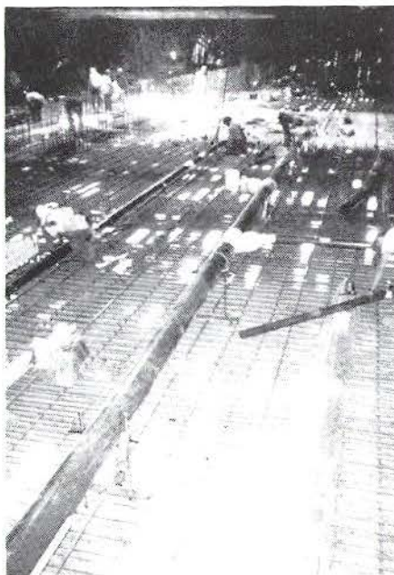
OVERVIEW OF THE REBAR PLACEMENT ACTIVITIES IN THE STATION'S SOUTHERN END (INVERTS 12 THRU 16)
