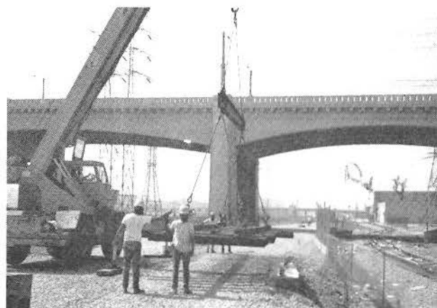
PLACING PREASSEMBLED SWITCH POINTS FOR NO. 8 SINGLE CROSSOVER AT 6TH ST. AREA
