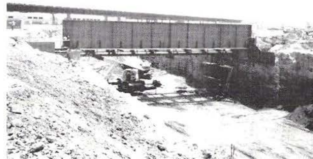
INSTALLATION OF PLATE GIRDERS FOR THE TEMPORARY VEHICLE BRIDGE
