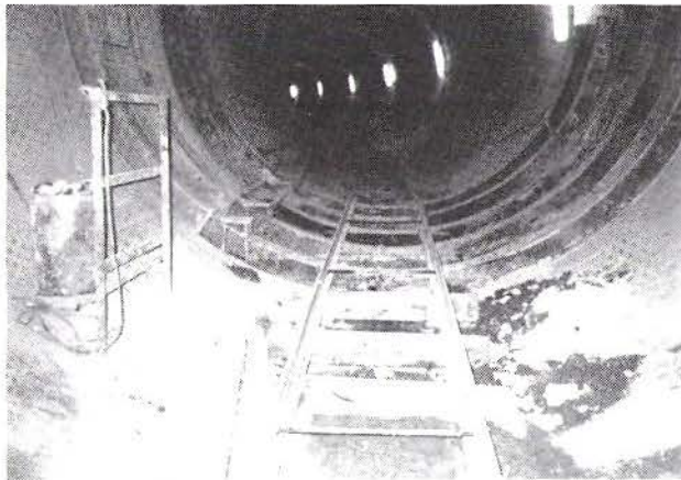
SUPPORT STEEL INSTALLED FOR CROSS PASSAGE BREAKOUT
