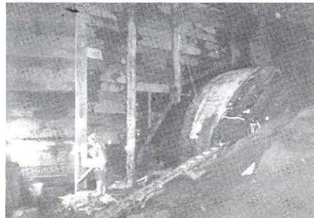
BREAKOUT OF AL TUNNEL INTO 5TH AND HILL STATION
