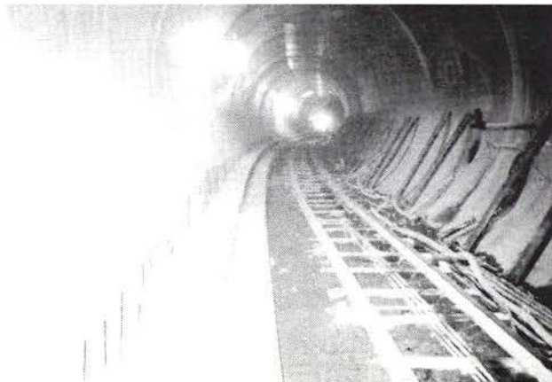
AL WALKWAY CONCRETE 1ST LIFT IN PLACE; FORMS ARE REMOVED STA 218+00 TO 210+50
