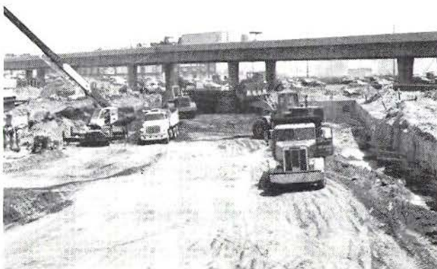
STRUCTURE EXCAVATION - NORTH END NEAR BUSWAY
