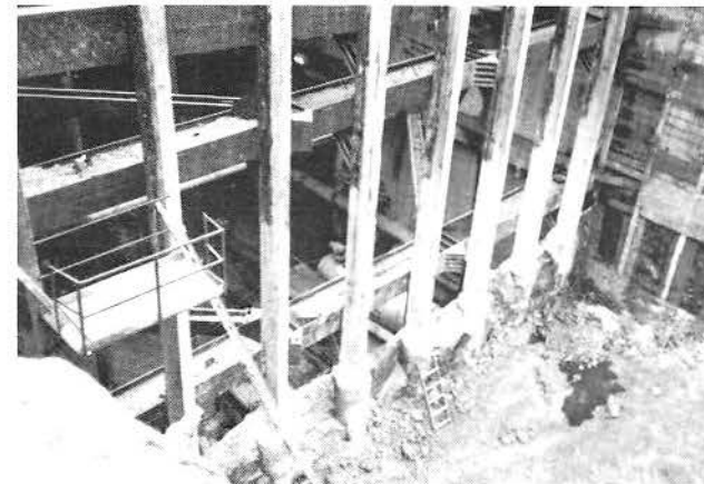
EXCAVATION AROUND SOLDIER PILES AT A171/A175 INTERFACE A RAIL CONCRETE AGITATOR CAR CAN BE SEEN AT INVERT GRADE OF A171 SHAFT
