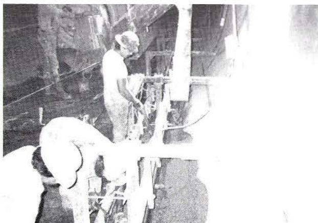
CONCRETE BEING PLACED IN AL WALKWAYS, 1ST LIFT
