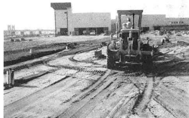
FINE GRADING SHOP TRACK MR-3 AND ROAD "C" (LOOKING SOUTH TOWARD MAIN SHOP BLDG.)
