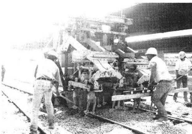
BALLAST TAMPING NEAR SOUTH END OF TEMPORARY RAILROAD TRESTLE
