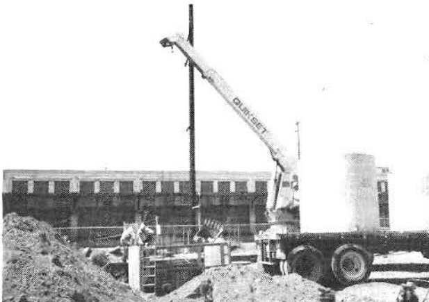
INSTALLATION OF SANITARY LIFT STATION HOUSING (LOOKING WEST TOWARDS SANTA FE AVE. FROM EAST OF SANITARY SEWER MANHOLE SS 7)
