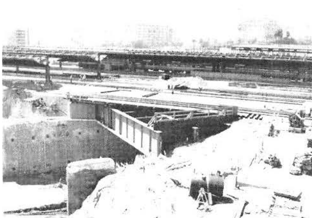
OVERVIEW OF TEMPORARY RAILROAD TRESTLE ACROSS STATION EXCAVATION IN LAUPT TRACKYARD
