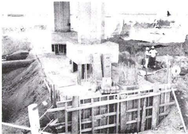
MUD SLAB FOR TRANSFER BEAM - UNDERPINNING BENT #4 BUSWAY
