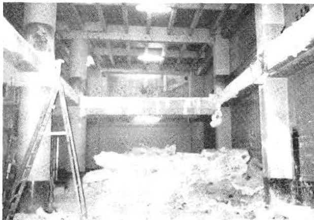
DEMOLITION OF SLABS FOR ENTRANCE TO STATION IN ROOSEVELT BUILDING - 7TH ST.
