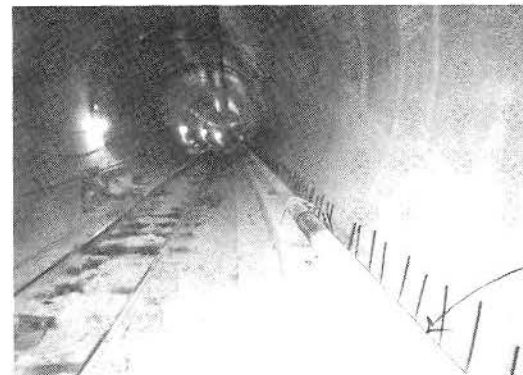
INSTALLATION OF WET STAND PIPE ON FIRST LIFT OF WALKWAY IN AR TUNNEL
