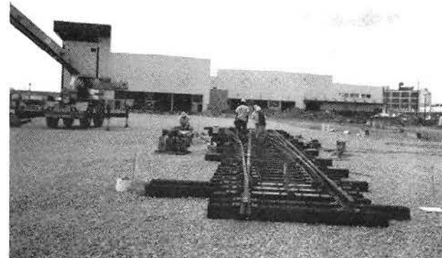
ASSEMBLING PRE-FABRICATED YARD TURNOUT NORTH OF MAIN SHOP BLDG. (LOOKING SOUTH TOWARDS MAIN SHOP BLDG.)
