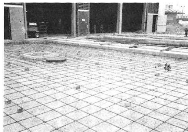
SERVICE & INSPECTION APPROACH APRON, READY FOR CONCRETE PLACEMENT
