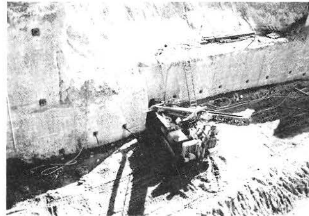
INSTALLATION OF TIEBACK ANCHOR TENDONS THRU SLURRY WALLS
