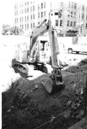
COMMENCING THE SOUTHEAST ENTRANCE EXCAVATION IN YARD I (SOUTHEAST CORNER OF 5TH/HILL ST.)
