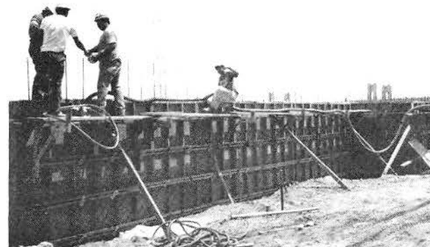
PUMPING CONCRETE FOR WEST WALL OF HEAVY CAR CLEANING PLATFORM (LOOKING SOUTHEAST FROM EAST SIDE OF MAIN SHOP BLDG.)
