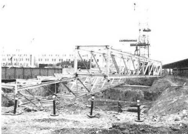
PLACING THE EAST PASSENGER BRIDGE ACROSS STATION EXCAVATION
