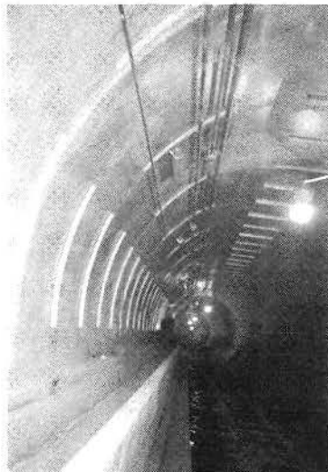
INSTALLATION OF ELECTRICAL CONDUITS IN AL TUNNEL
