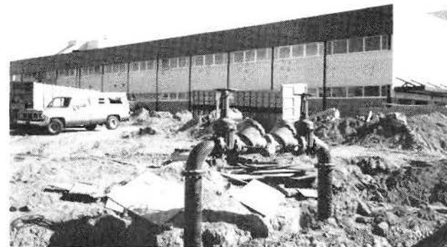
INSTALLATION OF 10" FIRE PROTECTION BACKFLOW PREVENTER CONNECTING TO CITY'S WM VAULT (LOOKING EAST TOWARDS WEST SIDE OF MAIN SHOP BLDG.)
