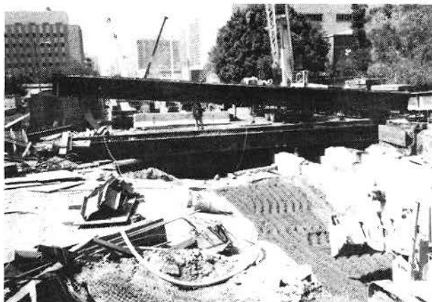
BACKFILLING ABOVE NORTH BLAST RELIEF SHAFT
