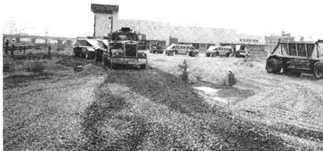
SPREADING BALLAST ON SHOP TRACKS NORTH OF MAIN SHOP BLDG. (LOOKING SOUTH TOWARDS MAIN SHOP BLDG.)
