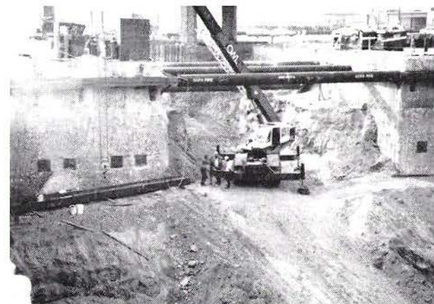
INSTALLING LATERAL BRACING ON SLURRY WALLS - NORTH PORTAL AREA
