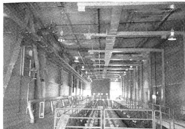
COMPLETED BLOWDOWN FACILITY
