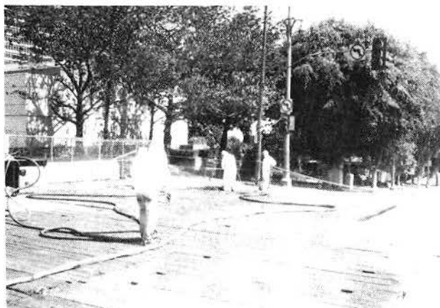
REAPPLYING NON-SKID COATING TO DECKING AT INTERSECTION OF FIRST & HILL STREETS
