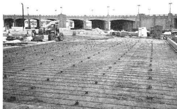
REBAR PLACED FOR APRON AT SOUTH END OF MAIN REPAIR AREA
