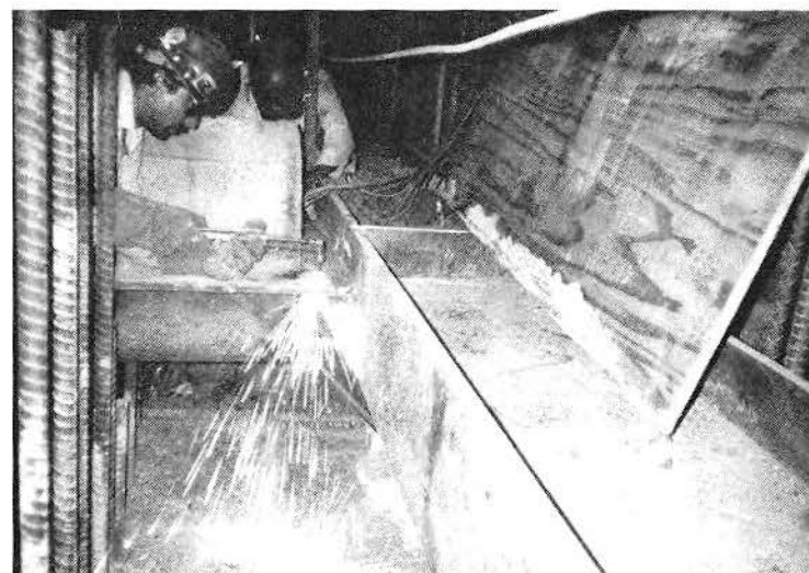
CUTTING "C" LEVEL WALER DURING TESTING OF STRUT REMOVAL PROCEDURE
