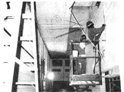
INSTALLATION OF CABLE TRAY SUPPORT, CORRIDOR #62 - RTD SPACE AT THE HOME SAVINGS BLDG.
