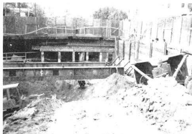
SOUTHEAST ENTRANCE EXCAVATION. EXCAVATION SUPPORT SYSTEM INSTALLATION
