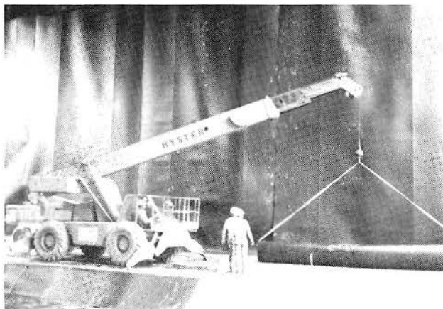
HDPE BEING ROLLED ALONG THE FACE OF THE NORTH SLURRY WALL, VIEW FACING NORTH WALL
