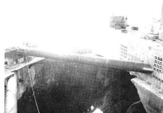
SEISMIC BRACE BEING INSTALLED ON TRANSFER BEAM
