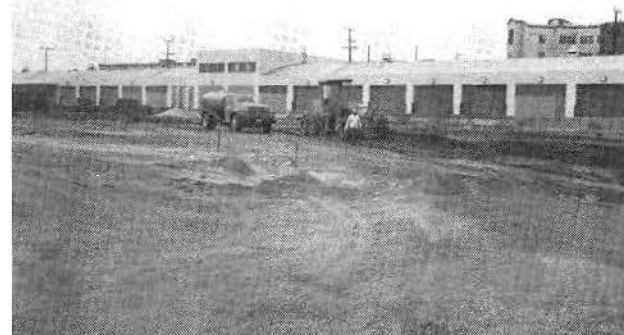
GRADING WORK FOR NON-ELECTRIFIED MAINTENANCE-OF-WAY AND OUTDOOR STORAGE TRACKS, EAST OF M.O.W. BLDG. (LOOKING SW TOWARDS M.O.W. BLDG.)
