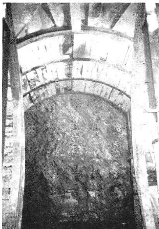
CROSS PASSAGE #4 AFTER COMPLETING 60% OF EXCAVATION FROM AR SIDE
