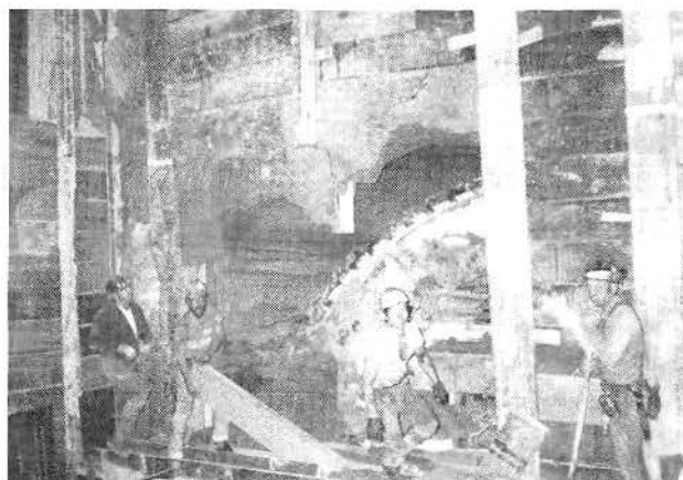
WORKMEN REMOVING SOLDIER PILES AND LAGGING AT BREAK THROUGH INTO EAST WALL OF A165 STATION
