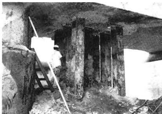
EXISTING BENT SUPPORT BEING REMOVED FROM TRANSFER BEAM
