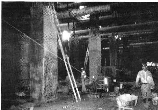
POURED STATION'S COLUMNS INVERT 13
