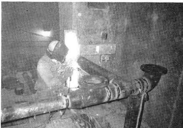
FABRICATION/INSTALLATION OF SUMP DISCHARGE PIPING
